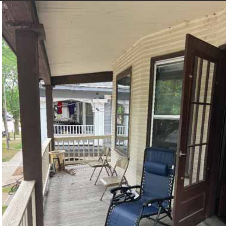
Photograph: 6 | 432/434 West Washington Avenue – Second Story Patio
