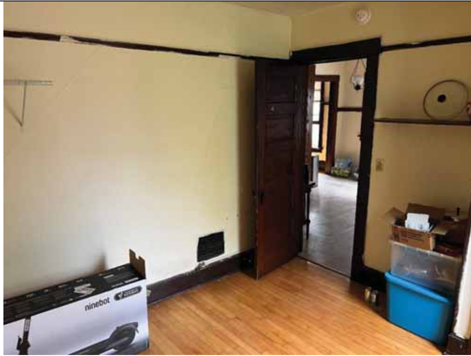
Photograph: 21 | 432/434 West Washington Avenue – Bedroom #1
