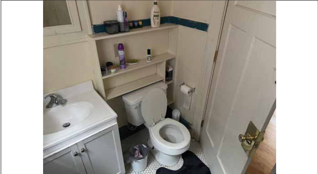
Photograph: 15 | 422/424 West Washington Avenue – Bathroom #2
