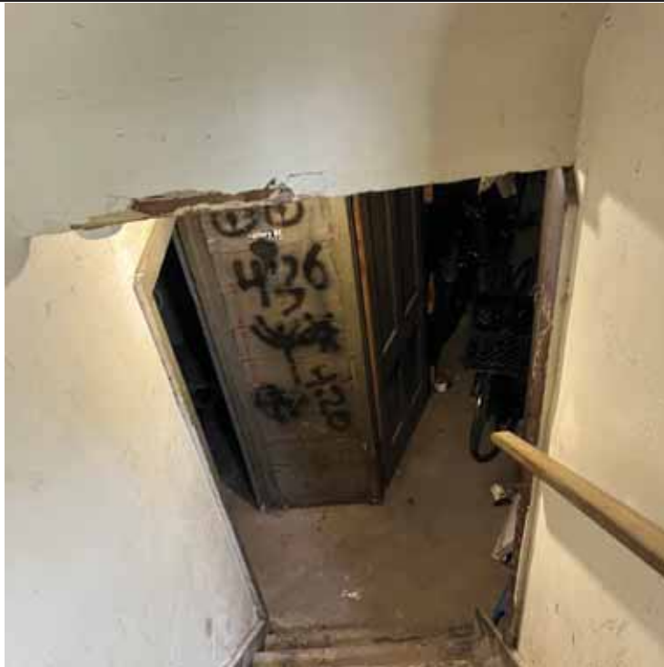
Photograph: 15 | 436/438 West Washington Avenue – Stairwell to Basement
