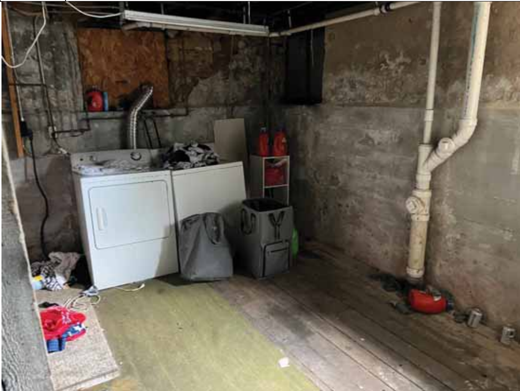
Photograph: 12 | 417 West Mifflin Street - Basement
