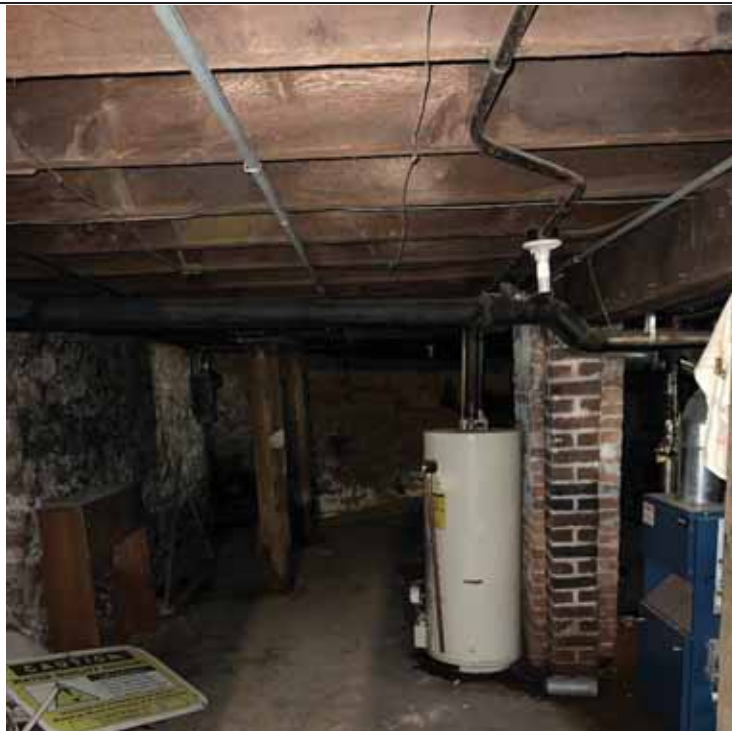
Photograph: 10 | 413 West Mifflin Street – Basement
