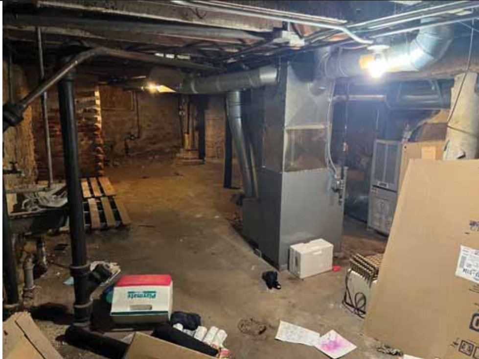
Photograph: 11 | 426 West Washington Avenue - Basement
