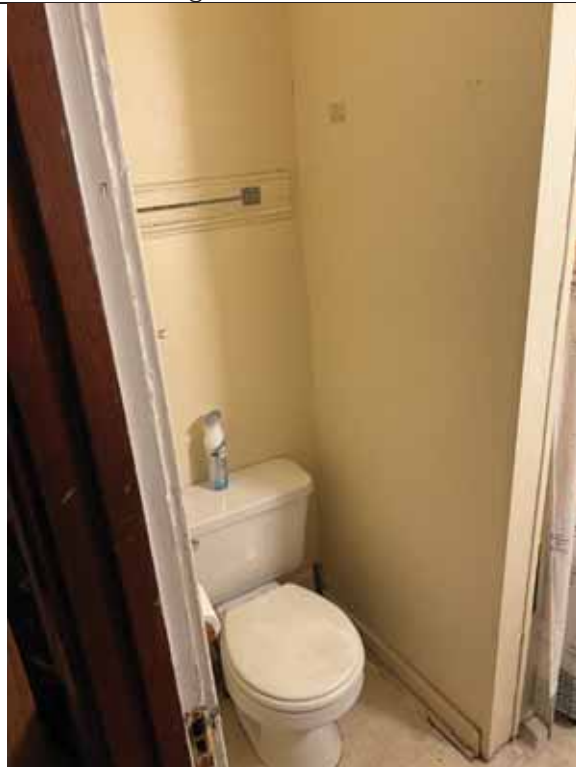
Photograph: 16 | 436/438 West Washington Avenue – Bathroom #1
