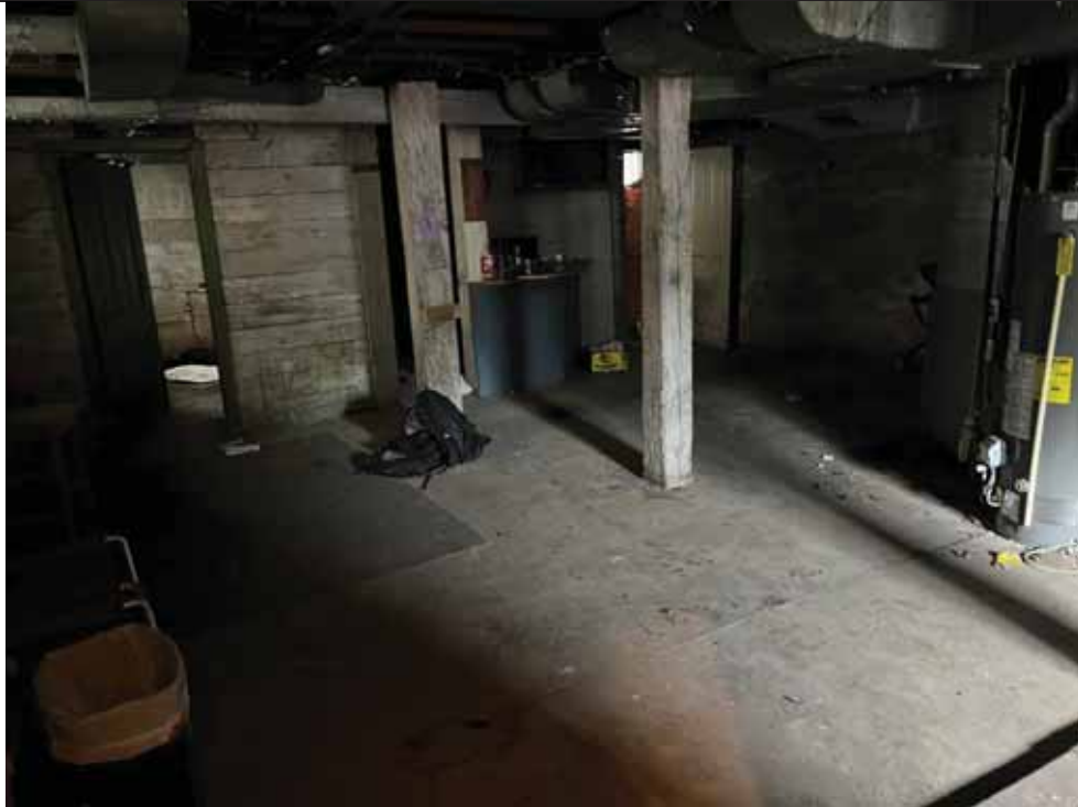
Photograph: 11 | 417 West Mifflin Street - Basement
