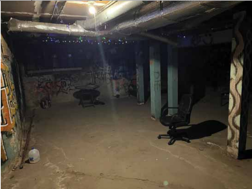
Photograph: 14 | 436/438 West Washington Avenue - Basement
