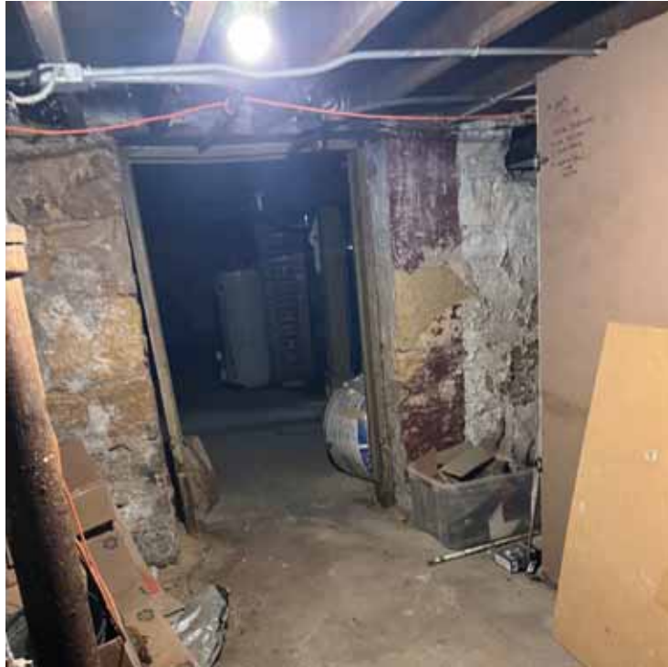
Photograph: 9 | 413 West Mifflin Street – Basement
