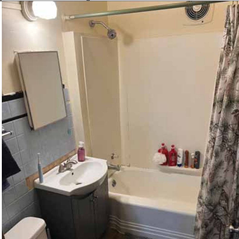
Photograph: 18 | 432/434 West Washington Avenue – Bathroom #1
