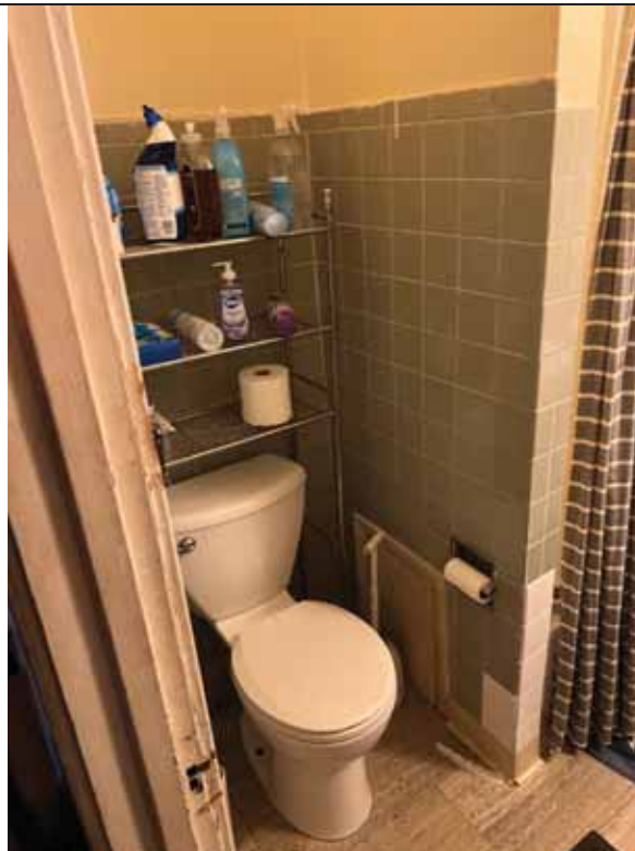
Photograph: 20 | 436/438 West Washington Avenue – Bathroom #3
