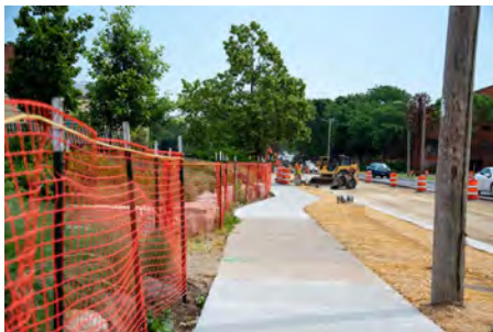
Small physical improvements example - sidewalk repair
