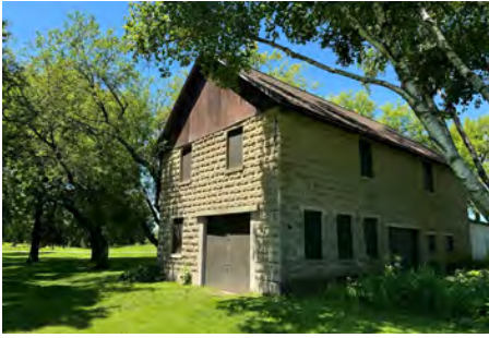
Amund Reindahl's barn, located in Reindahl park
