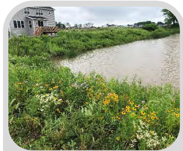
Saturn Drive Pond: a tier 1 wet detention pond.
