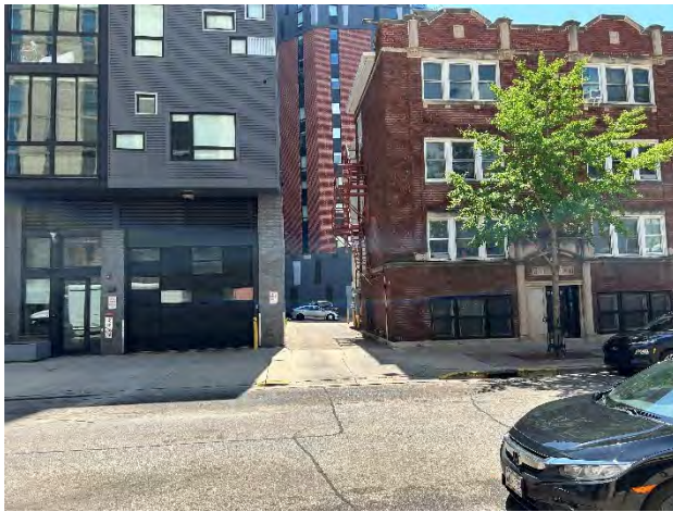
Gilman Street (view across street)
