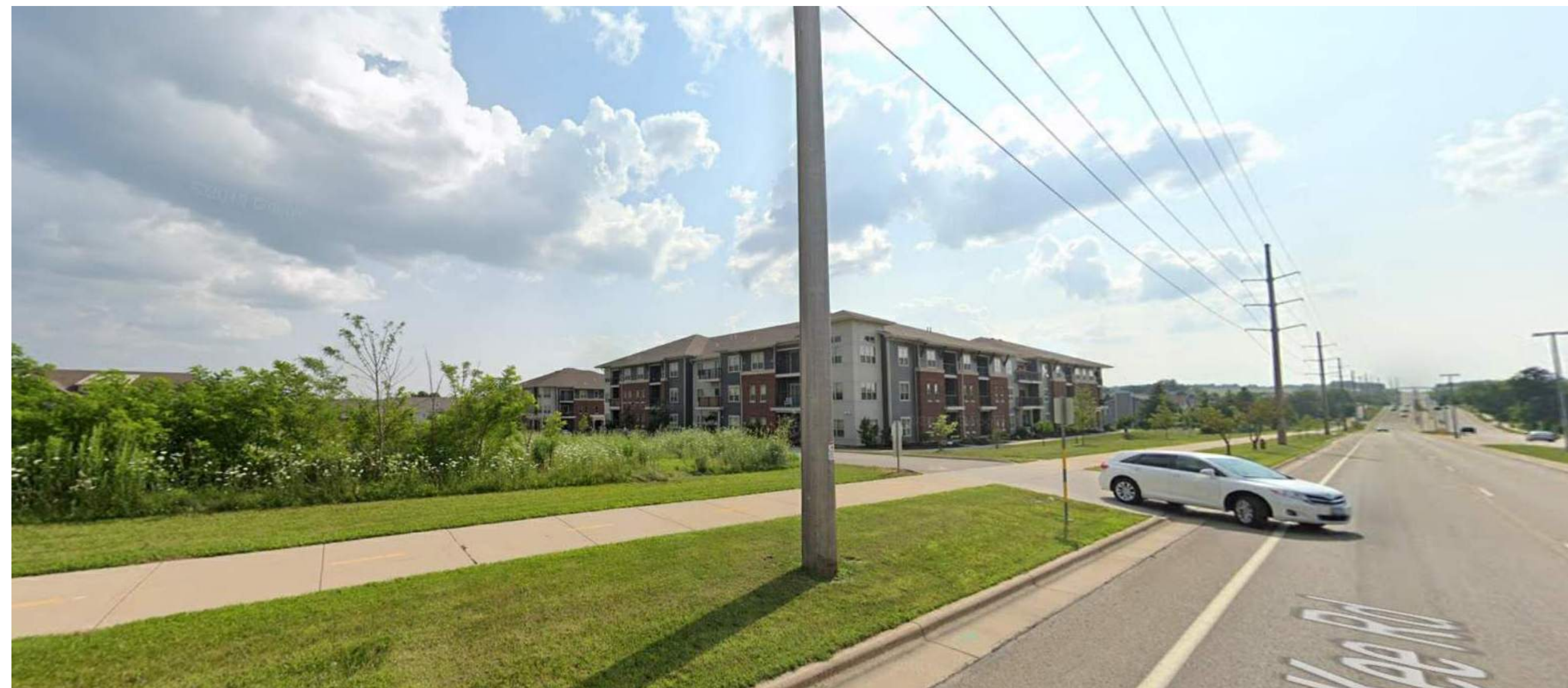
NORTHWEST CORNER - McKEE RD (LOOKING SOUTHWEST)
