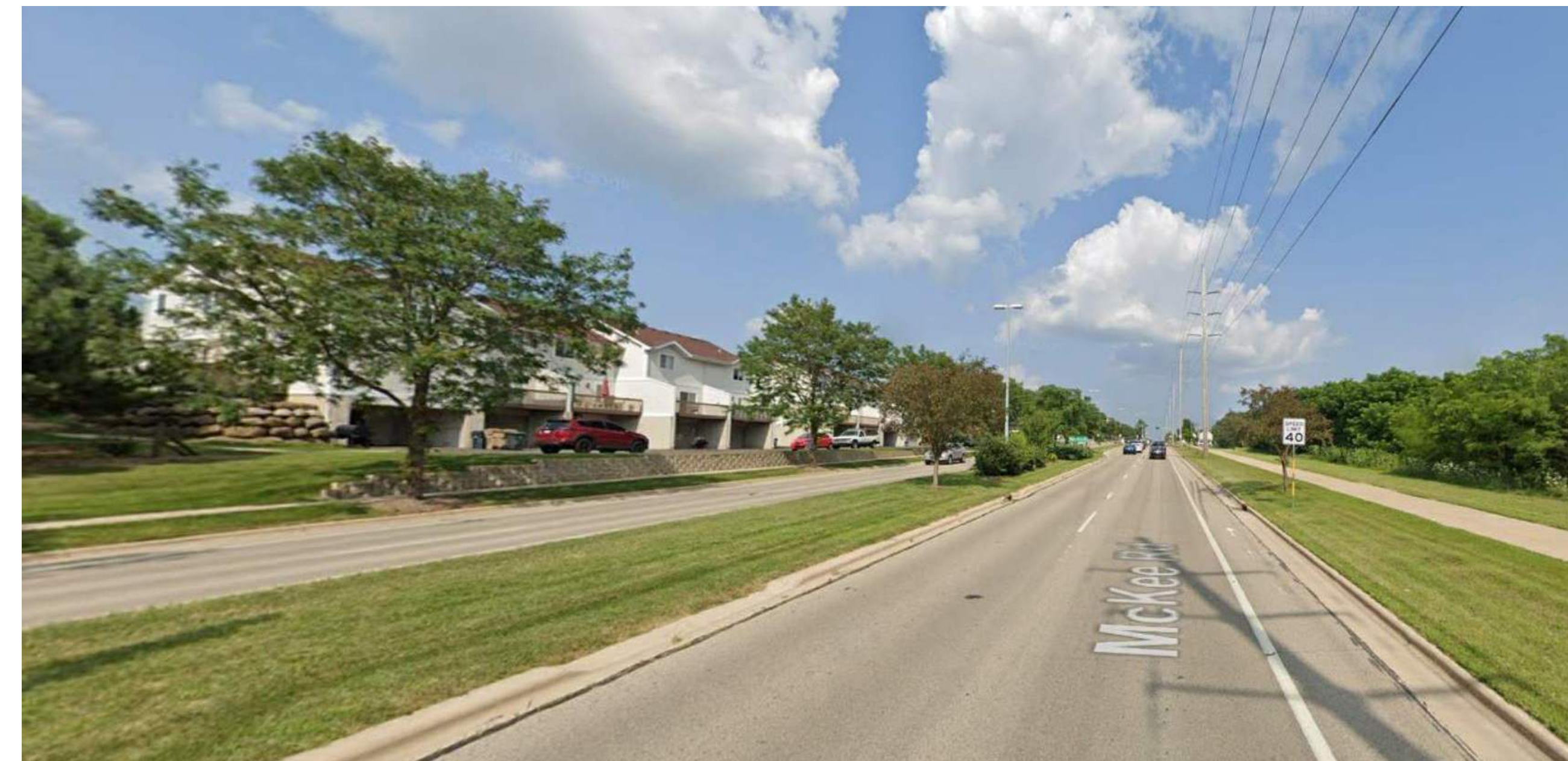
NORTHWEST CORNER - McKEE RD (LOOKING EAST)
