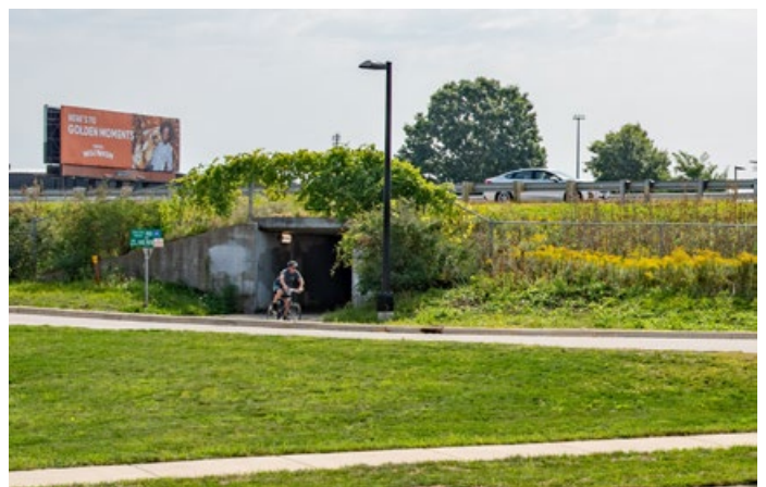
The Struck Street underpass of the Beltline is an important connection for pedestrians and bicyclists, but is in need of upgrades.
