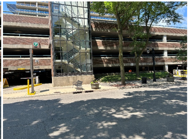
Frances Street (view across street)
