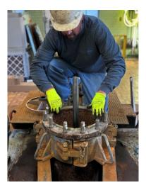
The maintenance crew of Matt Edgren, Dennis McCaslin, Joe Kennedy, Laine Kruizenga, and Kyle Rosemeyer re-stalled the parts and pieces of Unit Well 6 to repair a broken shaft. Pipe sections were stacked one on top of another until they reached a depth of 220 feet to reach the well level.
