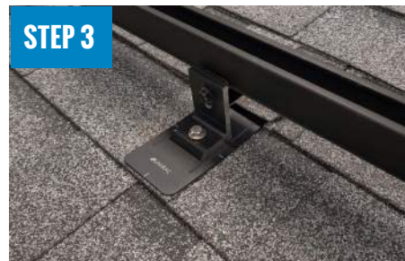
ATTACH L-FOOT TO RAIL
