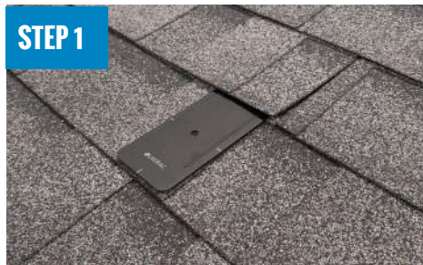
INSTALL FLASHKIT PRO SWITCHBLADE FLASHING
