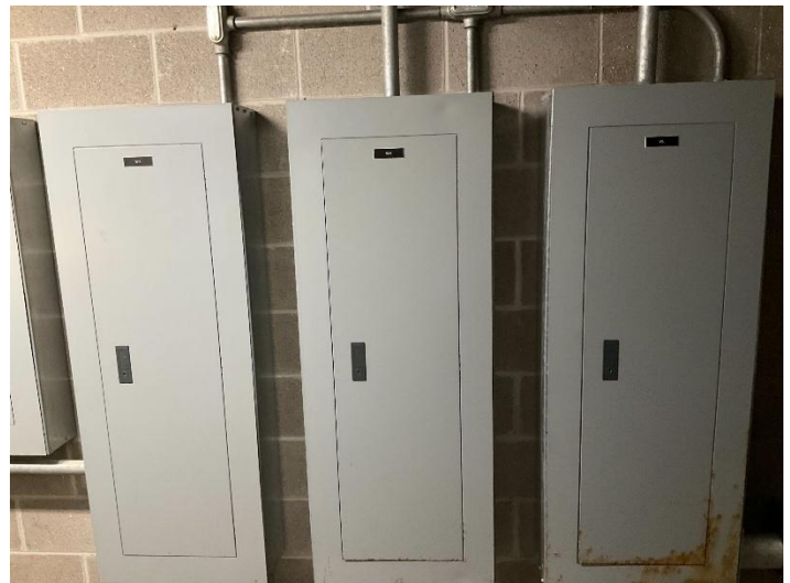
Existing Electrical Controls to be Replaced
