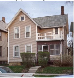
The applicant is proposing to remove the deteriorated enclosed porch and balcony and construct a simple covered porch and balcony design that is in keeping with the character of the district and of the structure. There are no historic photos to base the design upon, but it is similar in character to other historic resources in the vicinity and follows design precedent of previous approvals from the Landmarks Commission. The structure will feature wood
