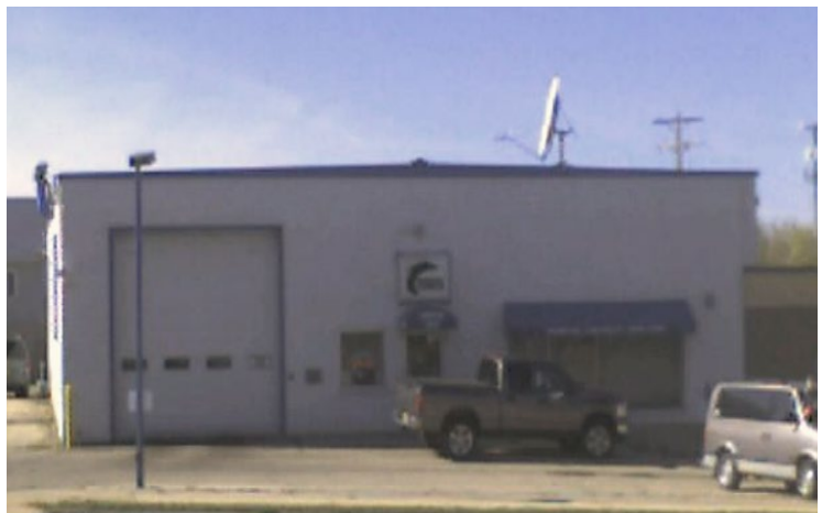
The Existing Park Street (East Elevation) Drawing- Image from City Assessor's Commercial Property Record.
