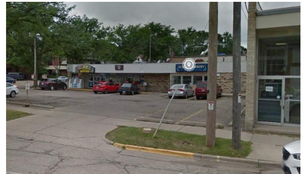
Winnebago Street Site Demolition Images
