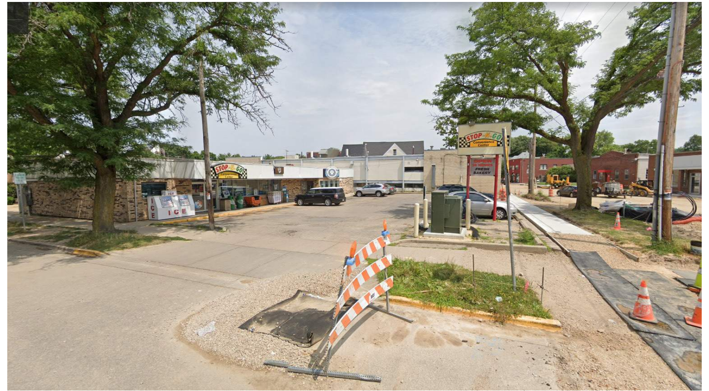
S 2nd Street Site Demolition Images
