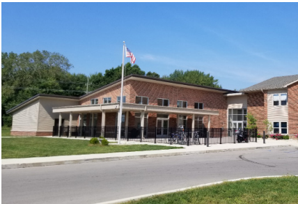
Chamber's Park Veterans Project
