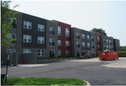
Enterprise Pointe - Under Construction
