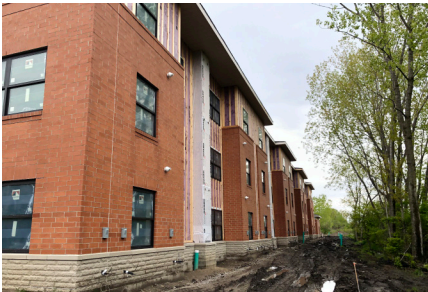
A Safe Haven - Under Construction
