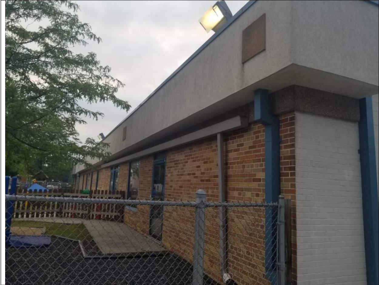
EXTERIOR NORTH ELEVATION
