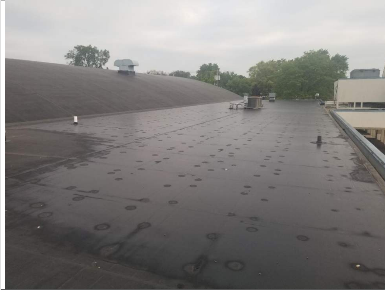
EXTERIOR ROOF EAST
