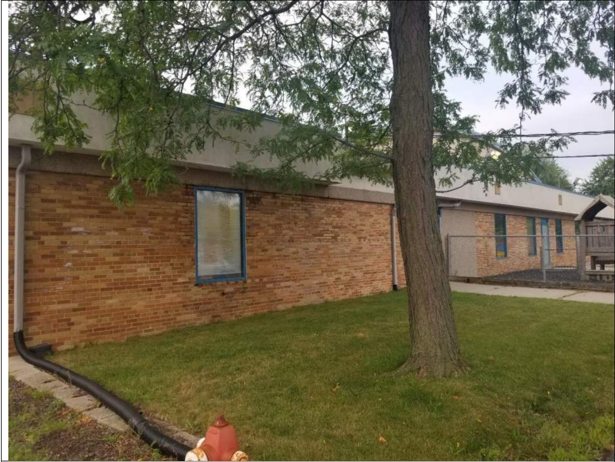
EXTERIOR NORTH ELEVATION
