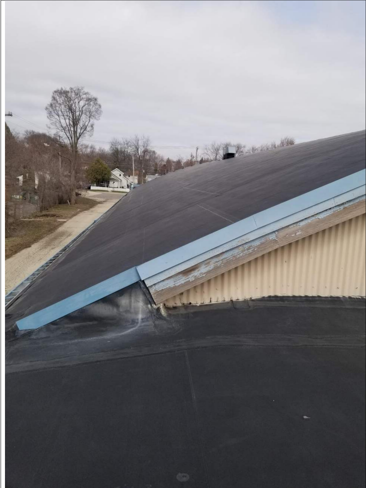
EXTERIOR ROOF WEST
