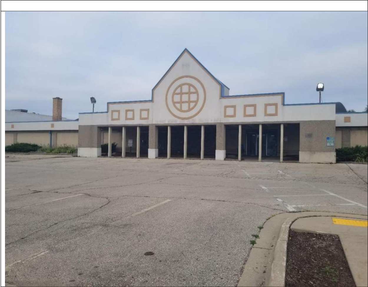
EXTERIOR EAST ELEVATON
