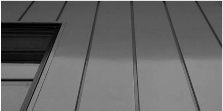
METAL PANEL 3: FLAT SEAM METAL PANEL w/ VERTICAL REGULAR PATTERN BASIS OF DESIGN ATAS VERSA-SEAM
