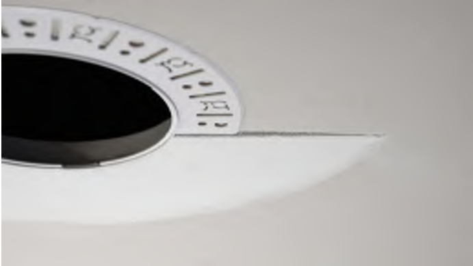
Partially finished mud ring, showing cross-section detail.
