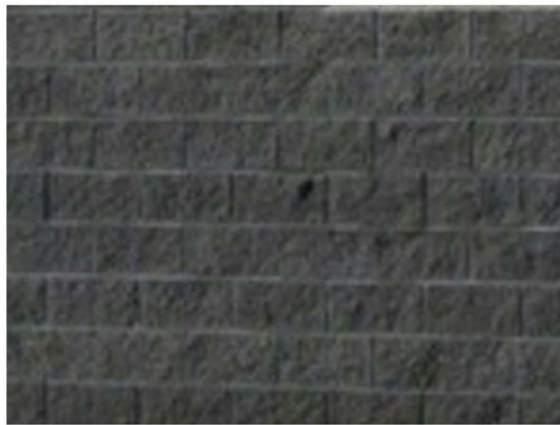
ROCK FACE CEMENT MASONRY BASE
