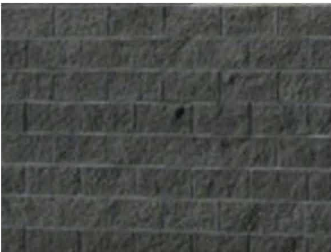
ROCK FACE CEMENT MASONRY BASE
