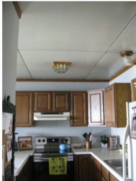
Kitchen – original ceiling
