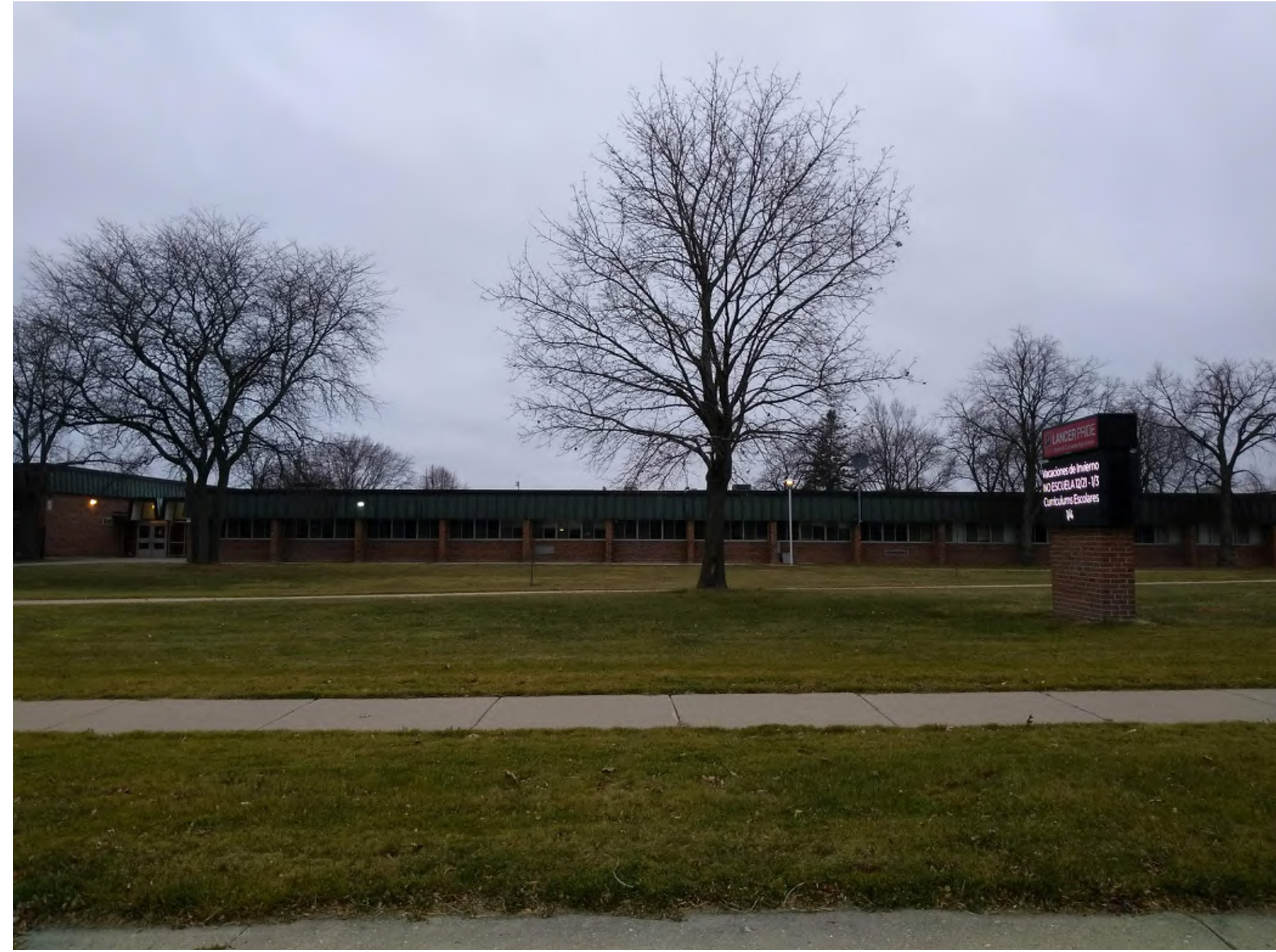
VIEW LOOKING NORTH FROM PFLAUM ROAD LOOKING AT PROPOSED NEW ENTRY LOCATION
