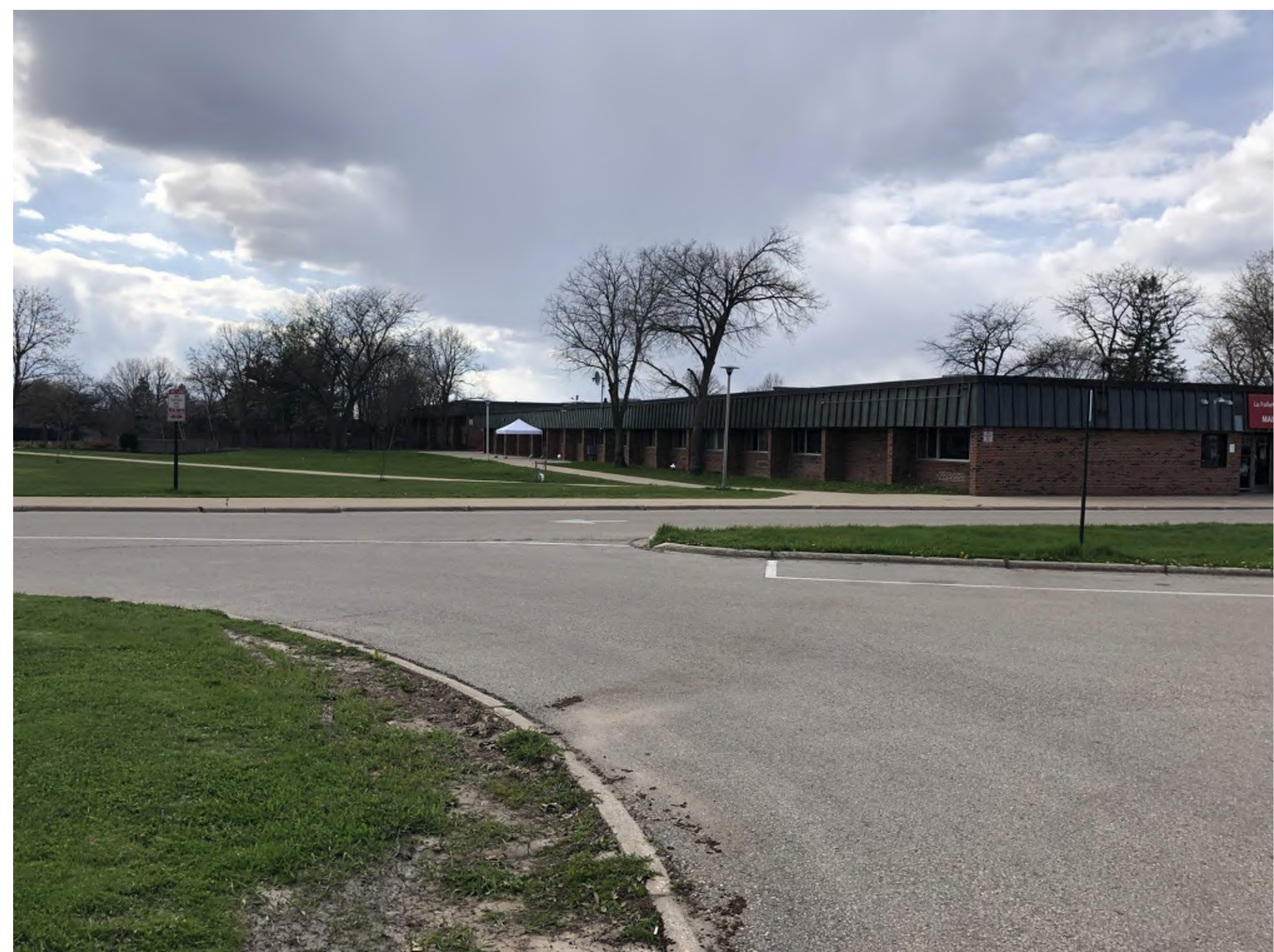
VIEW LOOKING NORTH WEST FROM PFLAUM ROAD LOOKING AT PROPOSED NEW ENTRY LOCATION
