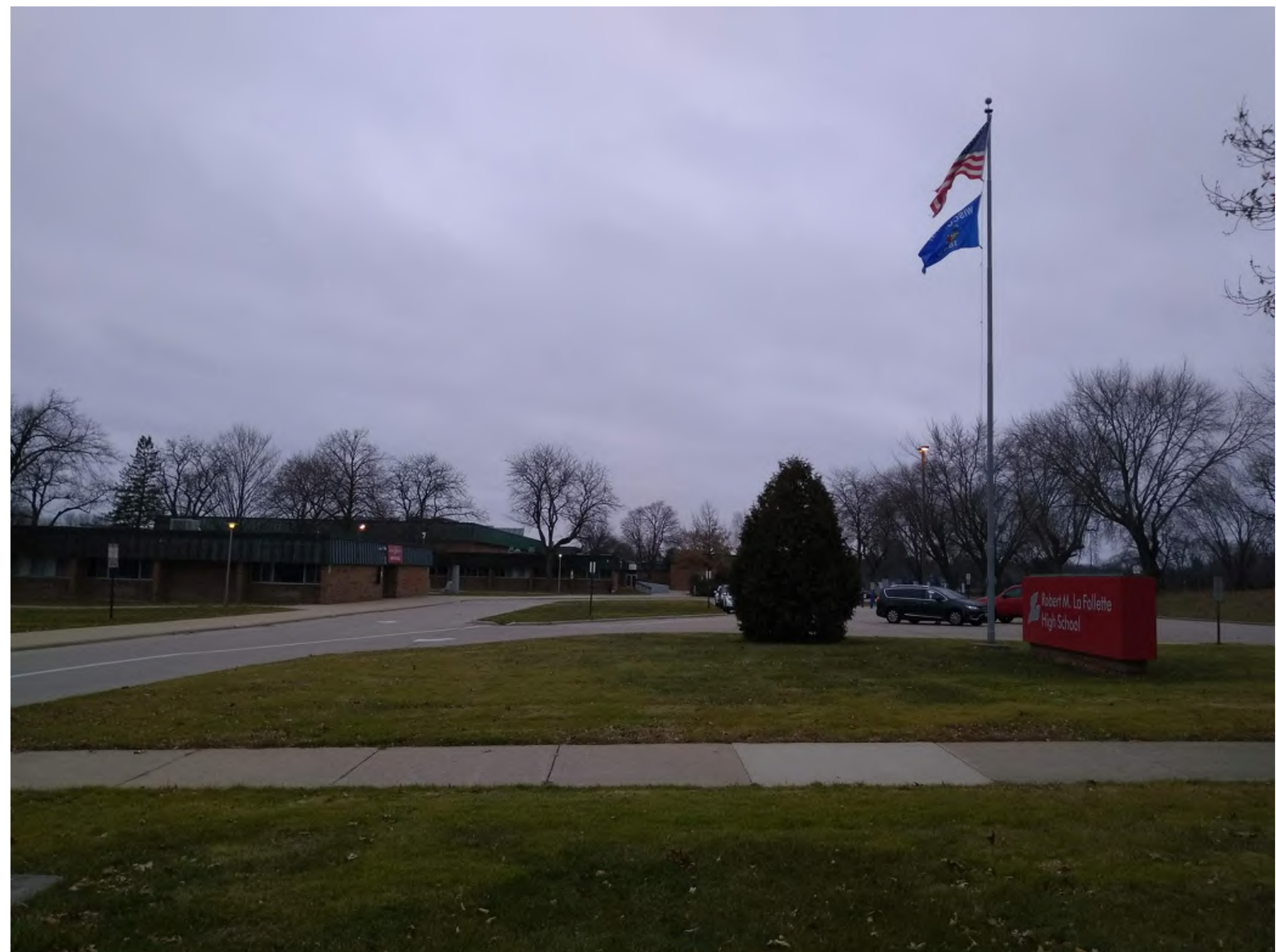
VIEW LOOKING NORTH FROM PFLAUM ROAD LOOKING AT PROPOSED FINE ART ADDITION LOCATION
