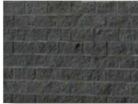
ROCK FACE CEMENT MASONRY BASE
