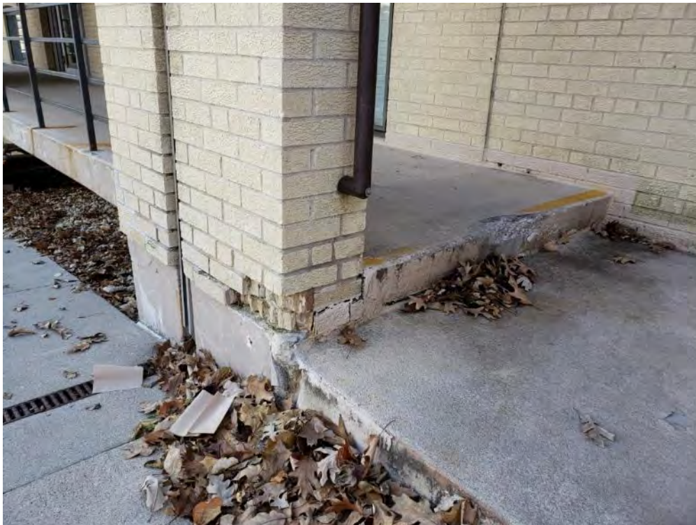
Masonry Pier 4 – damaged brick and foundation
