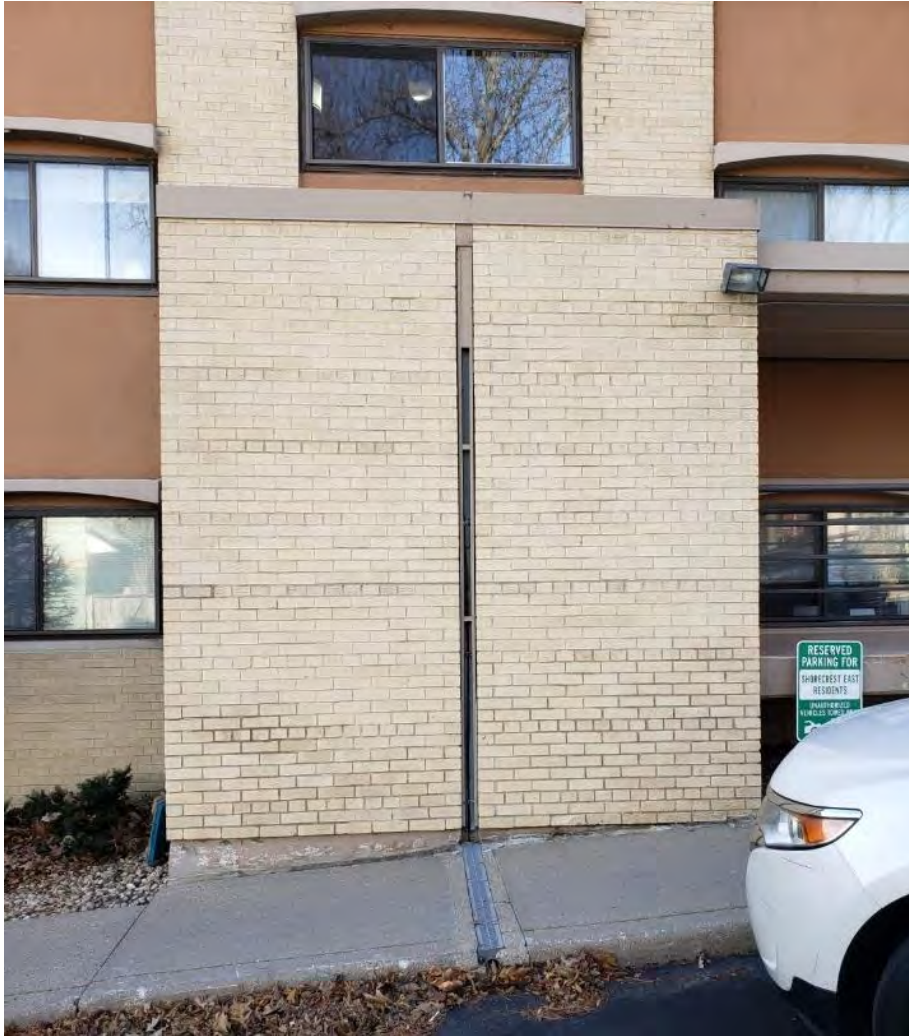
Masonry pier 3 – clean steel and attach new closure plate
