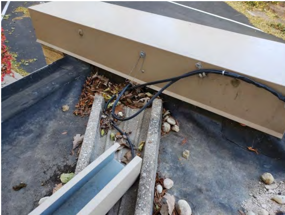
Downspout – Typical upper roof drainage onto walkway roof
