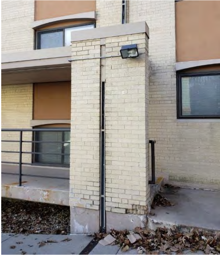
Masonry Pier 4 – damaged brick and foundation
