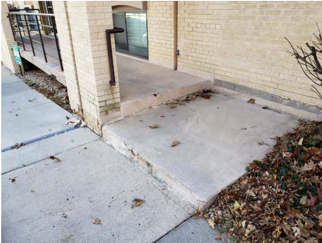
Masonry pier 2 – concrete steps in need of repair
