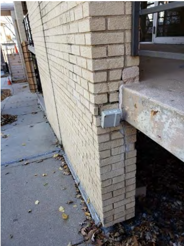
Masonry pier 5 – cracking in need of tuck pointing or replacement
