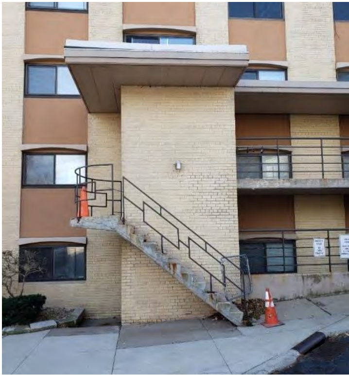
Precast deck damage – need for repair
