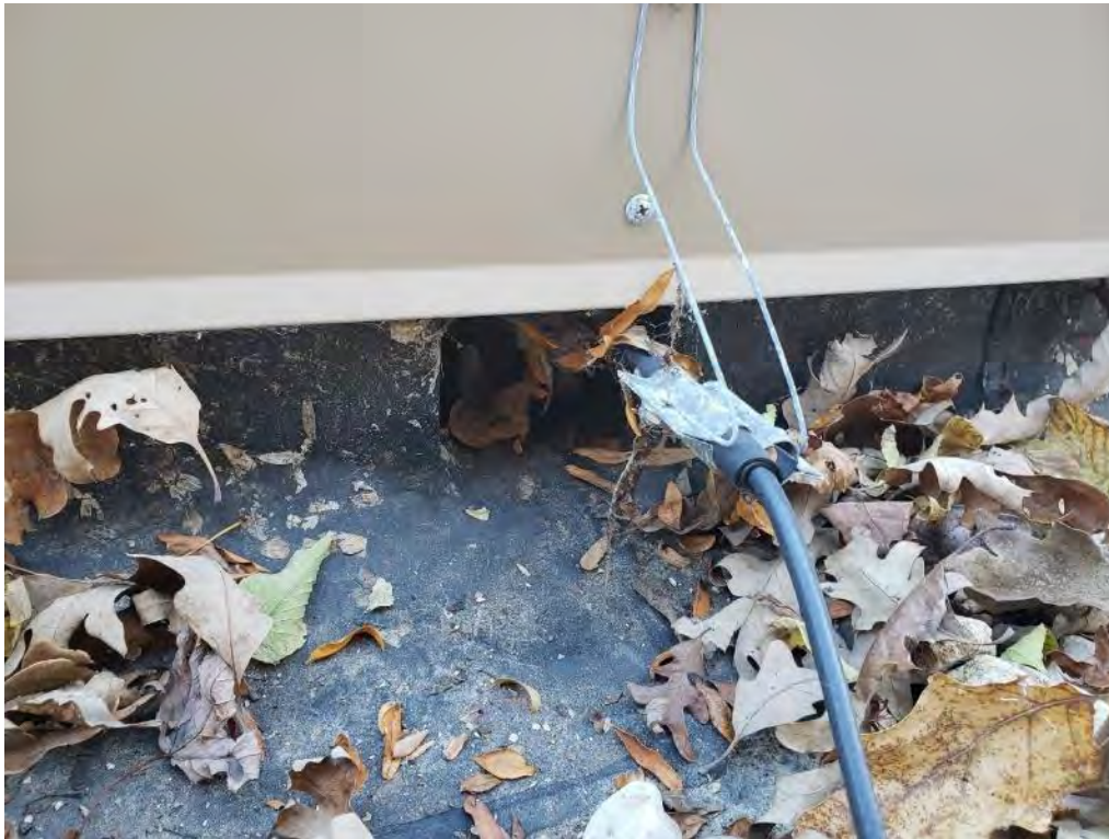
Downspout – Typical upper roof drainage onto walkway roof
