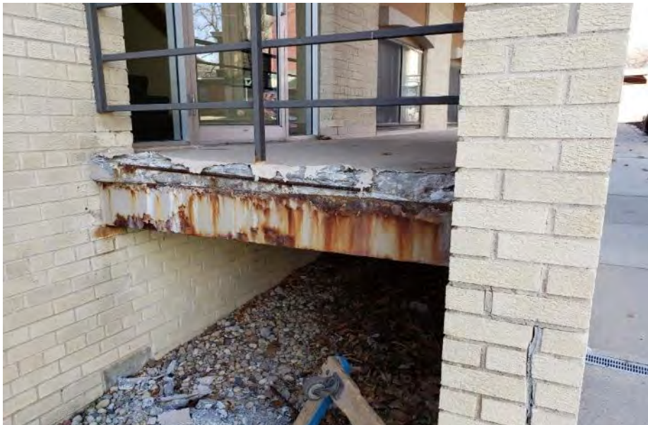
Masonry pier 3 – clean steel and attach new closure plate
