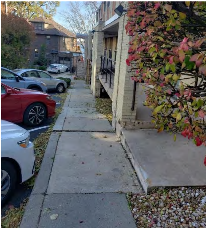
Concrete sidewalk – sloping towards building
