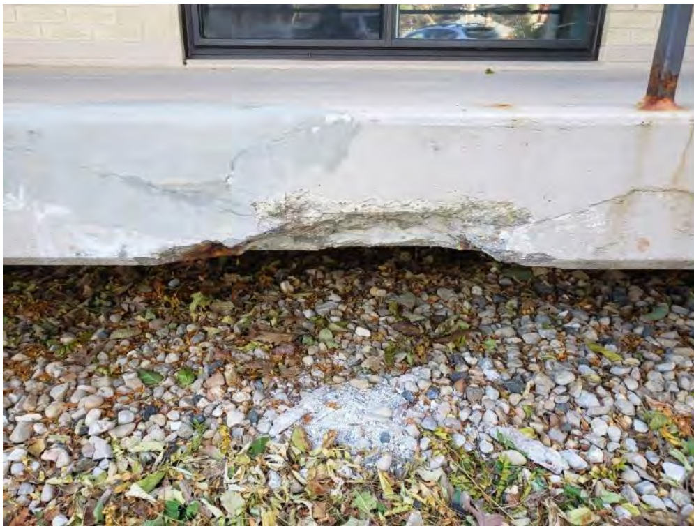
Precast deck damage – need for repair
