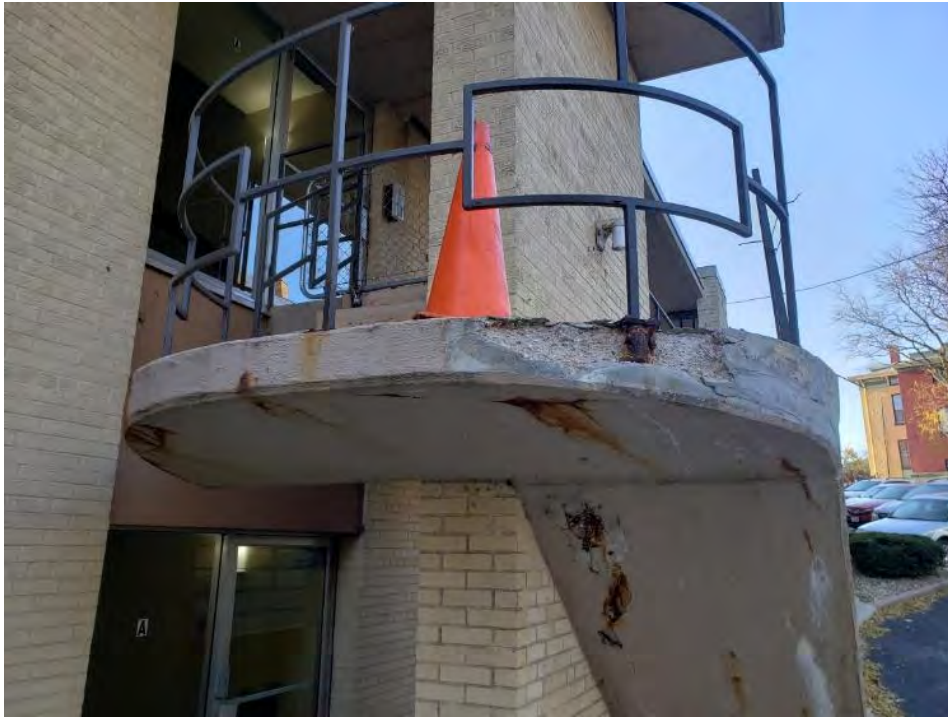
Concrete stair – spalling concrete and rusting rebar exposed
