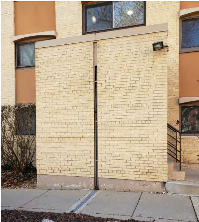
Masonry pier 1 – foundation repair and tuck pointing
