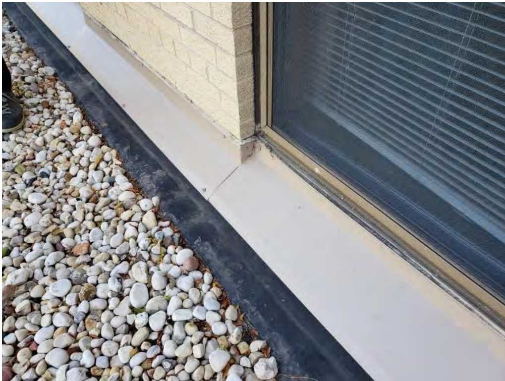
Roof flashing - roof to building connection appears sound
