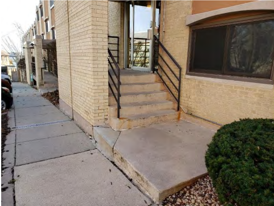
Concrete stoop and Masonry pier 1 – possible slab repair/replacement
