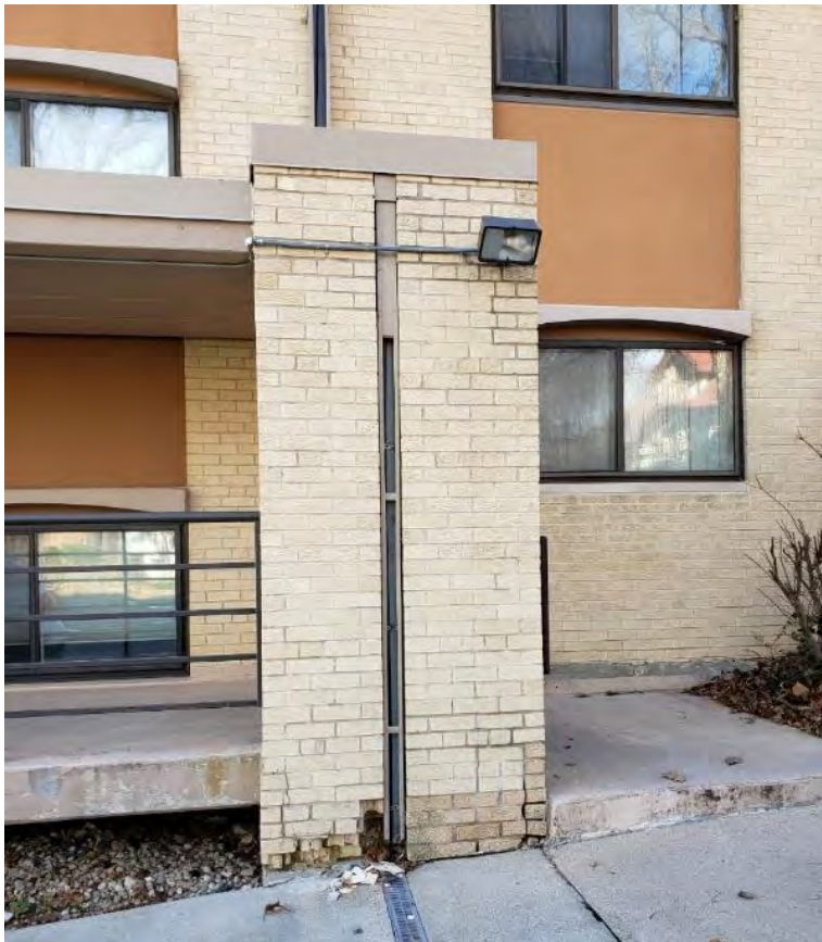
Masonry pier 2 - damaged base in need of replacement
