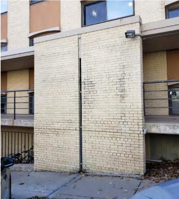
Masonry pier 5 – cracking in need of tuck pointing or replacement
