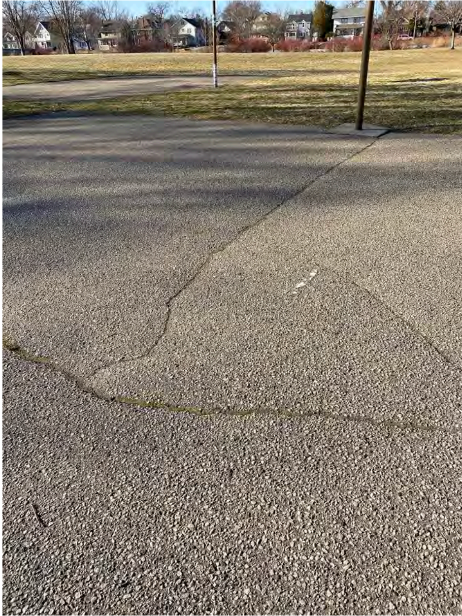
Asphalt contains large cracks
