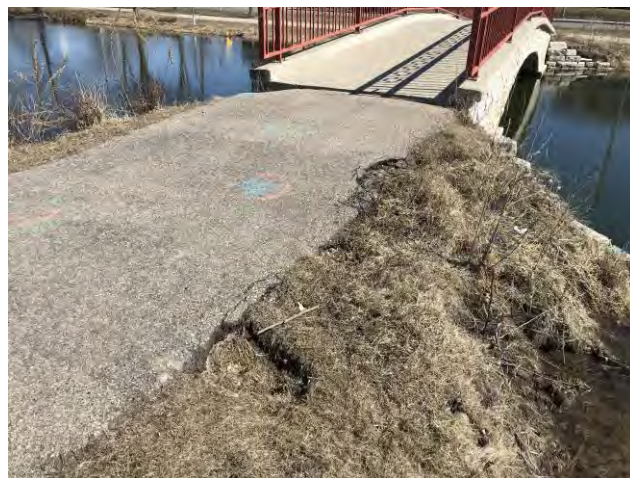
Figure 5–Path Damage and Settlement at North End of Bridge
