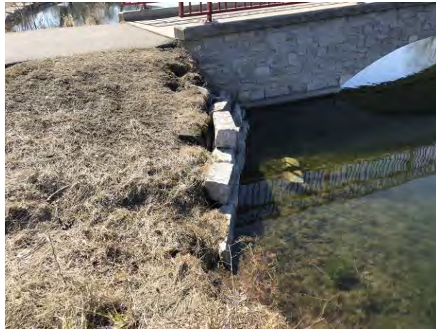
Figure 4–Typical Condition of Existing Wing Walls
