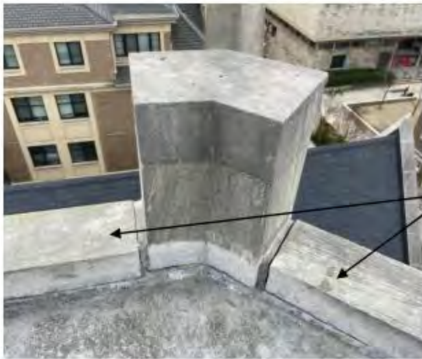
Loose stones at upper parapet. Stones will be removed and reset in mortar.
