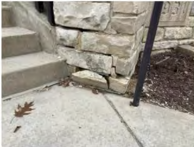
Loose stones at base of tower wall by sidewalk.
