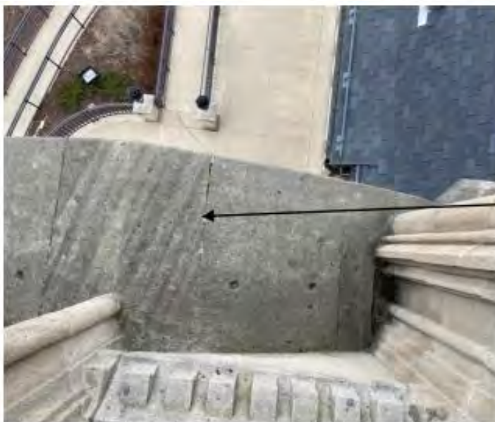
Recaulk sill joints.
