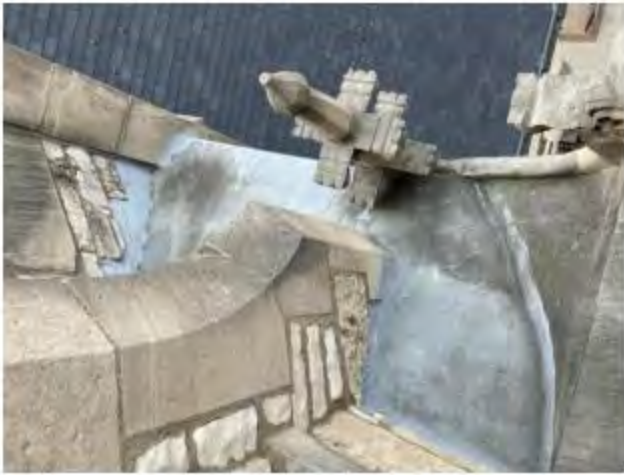
Deck coating on roof areas (8 roof locations total).
