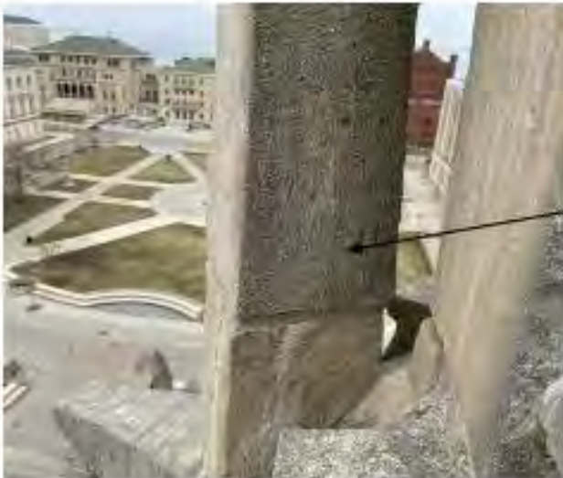
Rusted anchor with pediment cracked but still in place.
