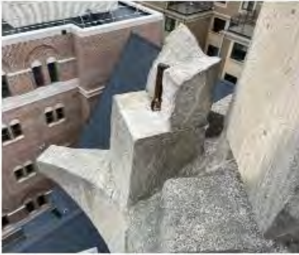
Rusted anchor with pediment removed.
