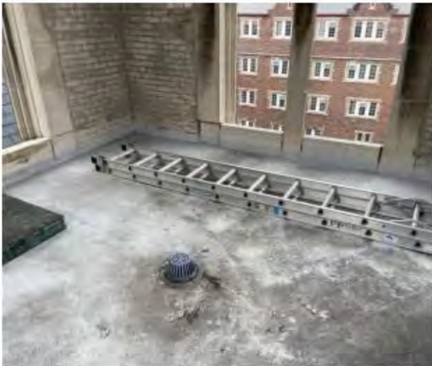
Deck coating on second exposed level.
