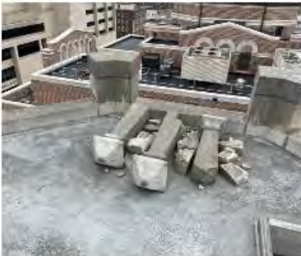
Three pediments removed and stored on upper roof.
