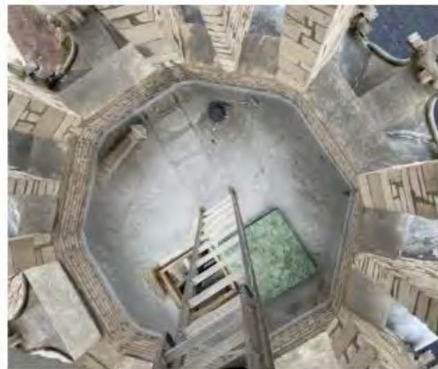
Deck coating on third exposed level
