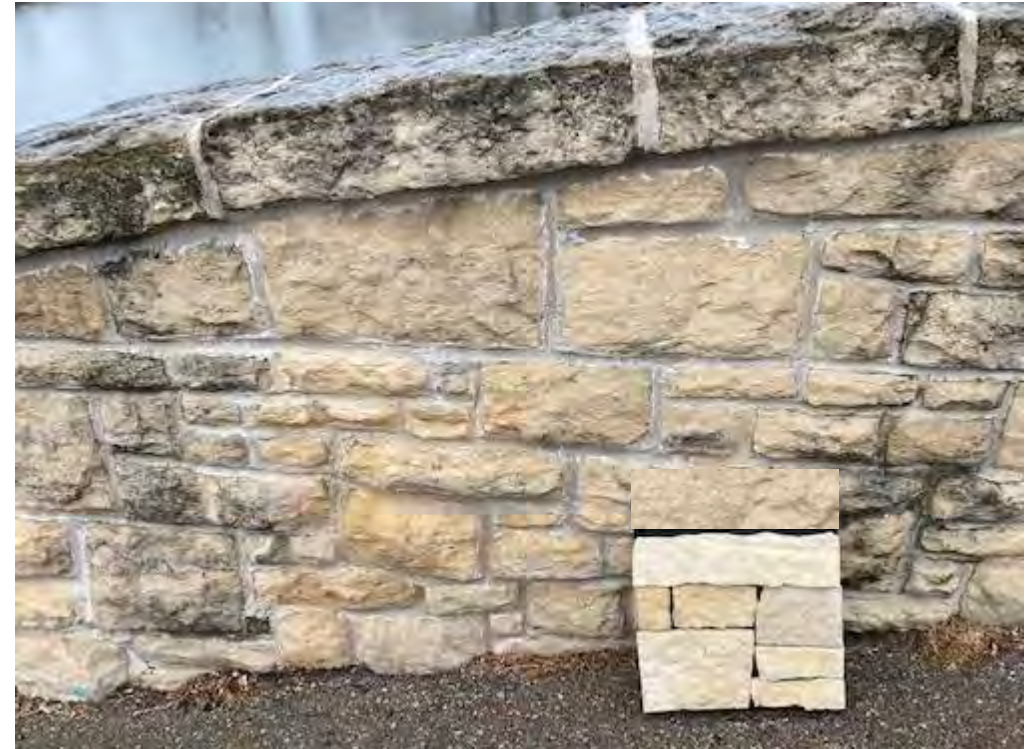
Kasota Stone Large ashlar pattern with flush mortar joints, slightly raked back, rock-face with natural split edges
