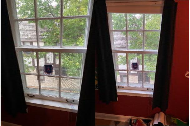
Given the condition of the existing windows, we believe that a replacement is the most feasible solution. The new replacement windows will be Pella Architectural Series and will be very similar in style to the existing windows. The replacement windows will be the same size as existing. The window specifications are attached to this submittal for your review.
