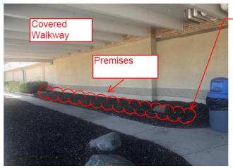
Location of posts for Wall-set back from Building facade, so when Wall is attached to posts it does not obstruct the sidewalk. Also, Wall should be set back roughly 3' from door to the right so it does not obstruct access. Premises=8' tall by 28' wide in this area.
