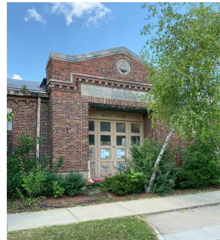
Wisconsin Telephone Co. Building
