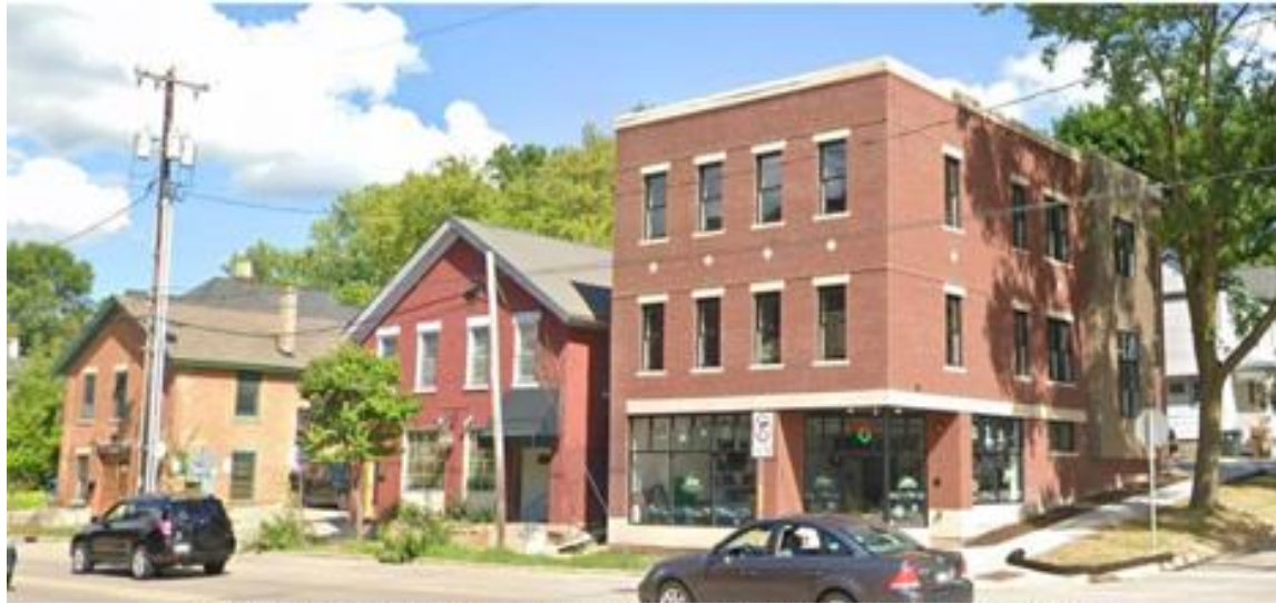
Streetview of 803-811 Williamson Street illustrating a similar street façade height
