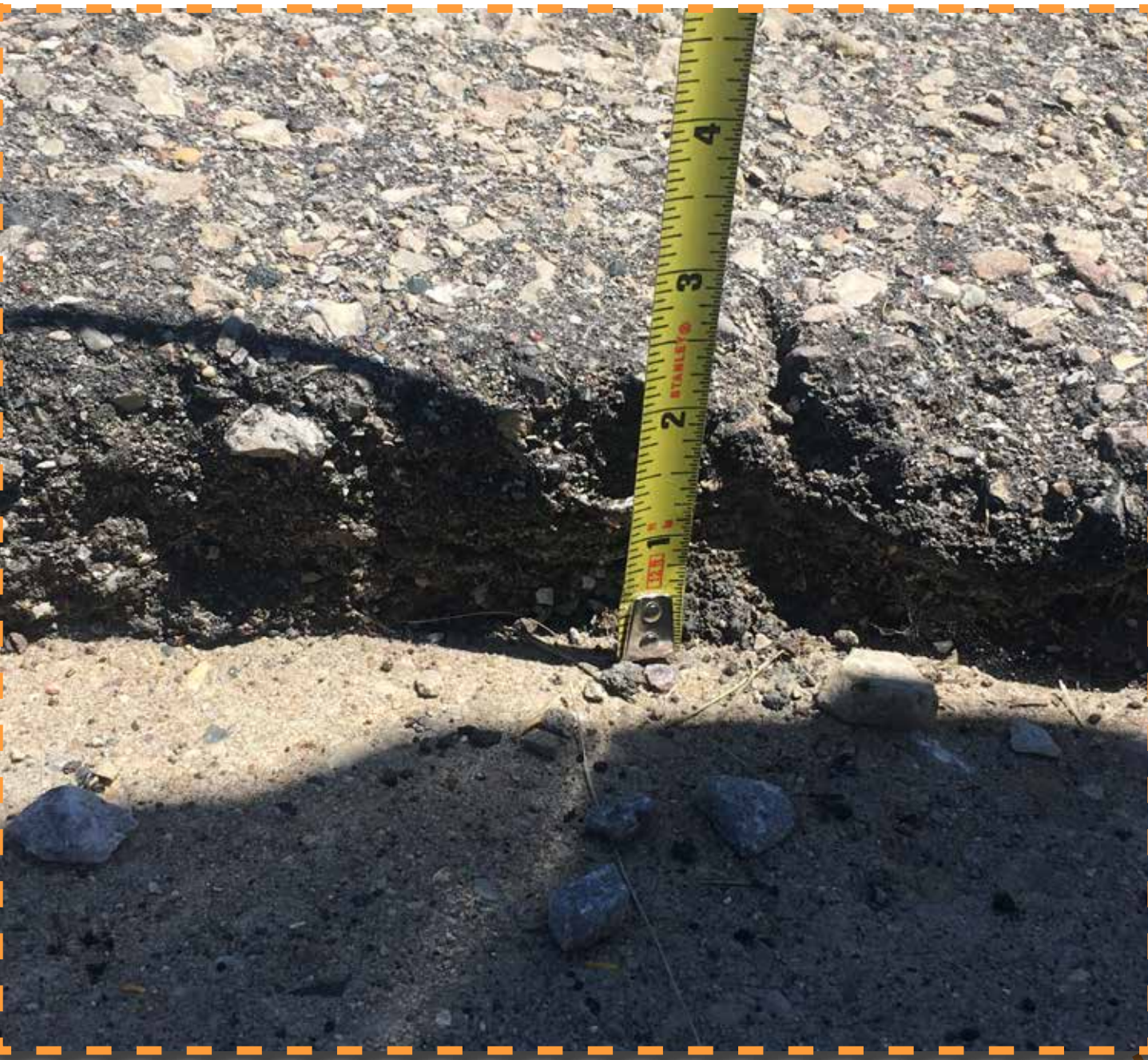
IMAGE 2/3: NON COMPLIANT ADA SIDEWALK AT TRACKS
