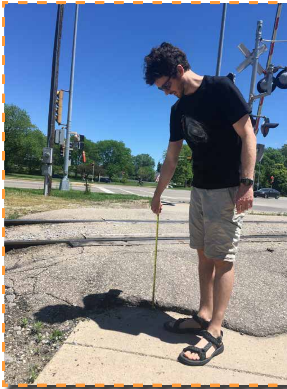
IMAGE 2/3: NON COMPLIANT ADA SIDEWALK AT TRACKS
