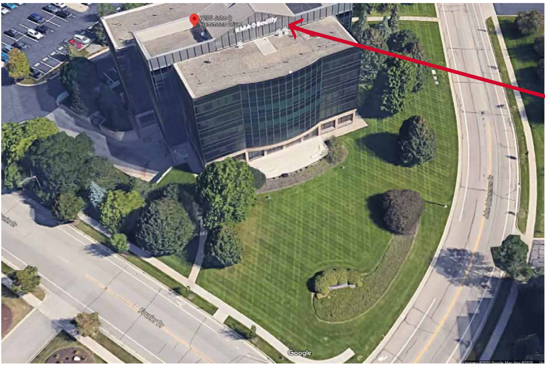
IMAGE BELOW IS OVERHEAD VIEW OF BUILDING
