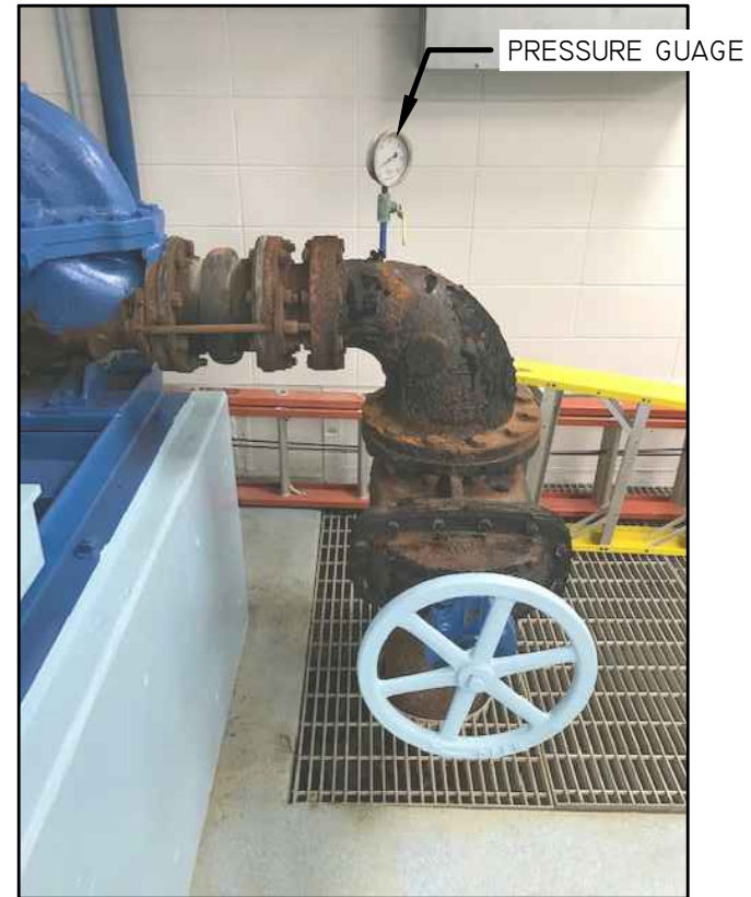
BOOSTER PUMP #1 SUCTION PIPE
