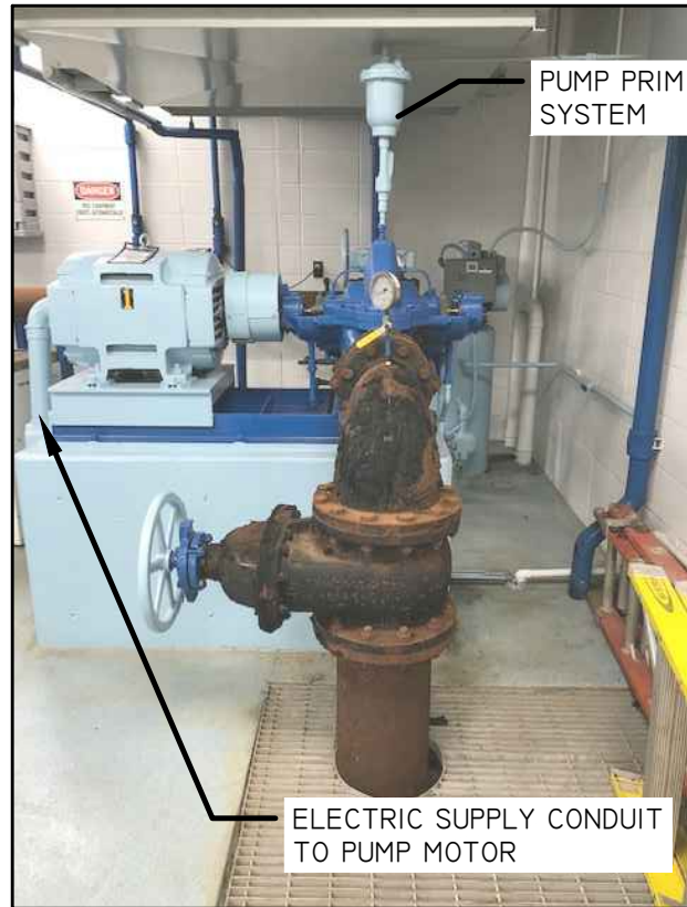
BOOSTER PUMP #1 SIDE VIEW
