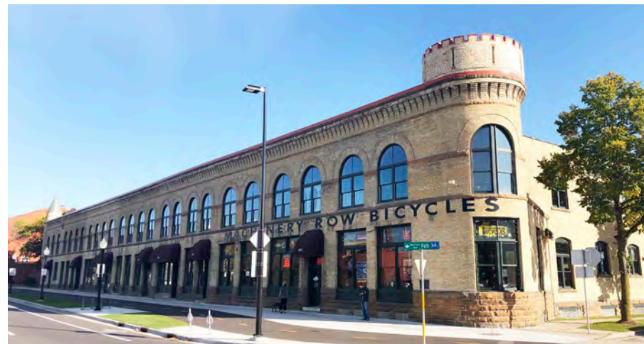
Machinery Row, 601-627 Williamson Street
