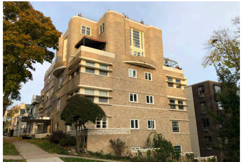
Quisling Towers Apartments, 1 East Gilman Street
