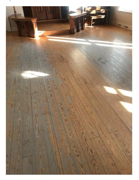
Gates of Heaven was constructed in 1863 and was relocated from West Washington Avenue to its current location in the early 1970s. During relocation, the original flooring was removed. The existing non-original flooring is 5 ¼" wide select pine with very few knots.
