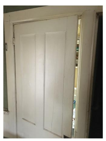
Fig. 14: Detail of solid, 4-panel interior door and casing, leading to bathroom.
