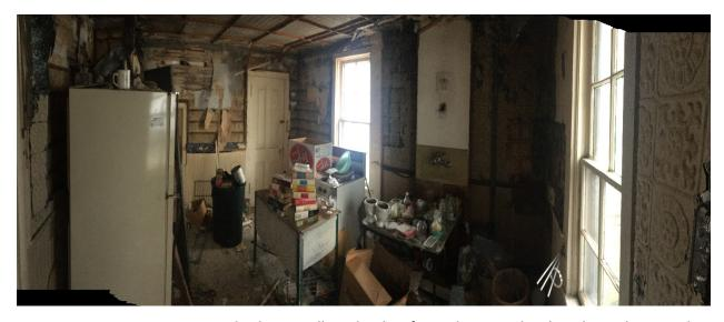
Fig. 16: Interior panoramic view, kitchen. Walls and ceiling formerly covered with embossed tin panels, now mostly removed to expose plaster and wood lath walls.
