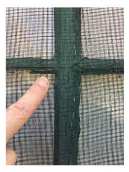
Fig. 11: Muntin detail on window, showing wider vertical member.
