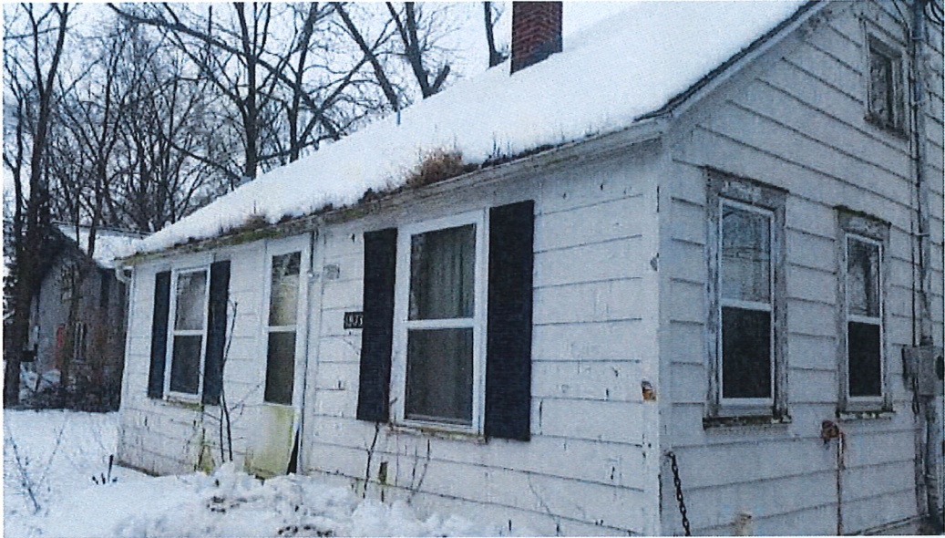
House at 4933 Femrite Drive
