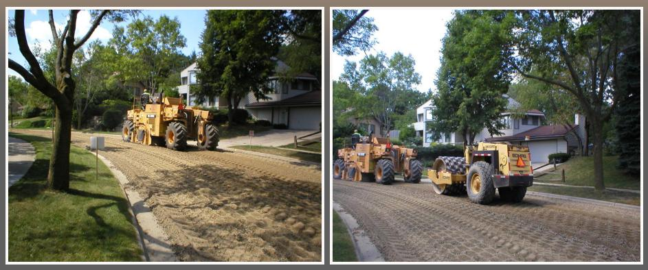
ASPHALT AND GRAVEL BASE ARE PULVERIZED
