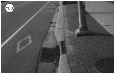
Where space is tight but drainage requirements dictate an 18 in. (0.45 m) drain, a special 1 ft. (0.3 m) curbhead may be used with a 1 ft. (0.3 m) gutter pan (fig. 3-13).
