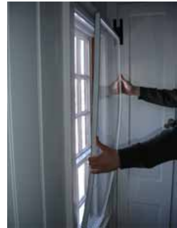
Interior storm panel.
