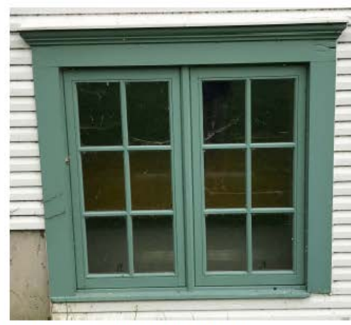
Window 10: Casement pair Change to 2 horizontal muntins at each sash. Replace/repair sill and jamb trim. Head trim to remain.
