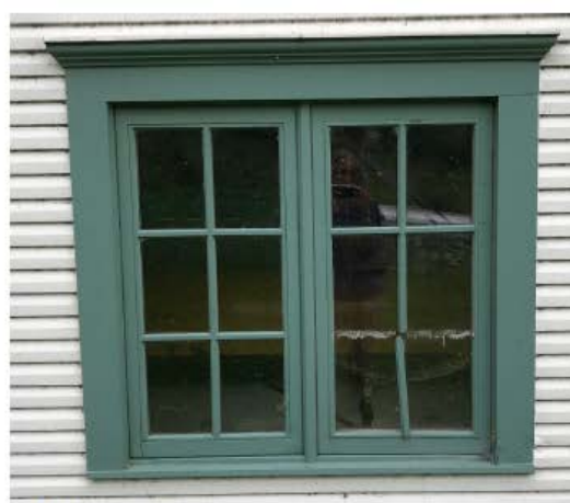
Window 9: Casement pair Change to 2 horizontal muntins at each sash. Replace sill and replace/repair jamb trim. Head trim to remain.
