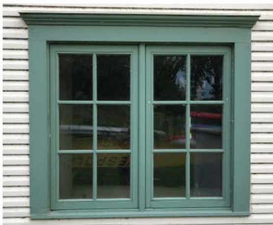
Window 8: Casement pair Change to 2 horizontal muntins at each sash. Repair sill and jamb trim. Head trim to remain.
