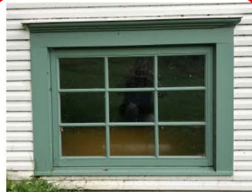
Window 11: Casement pair 1 horizontal muntin at each sash to match taller sash with two horizontal muntins. Replace/repair sill and jamb trim. head trim to remain.
