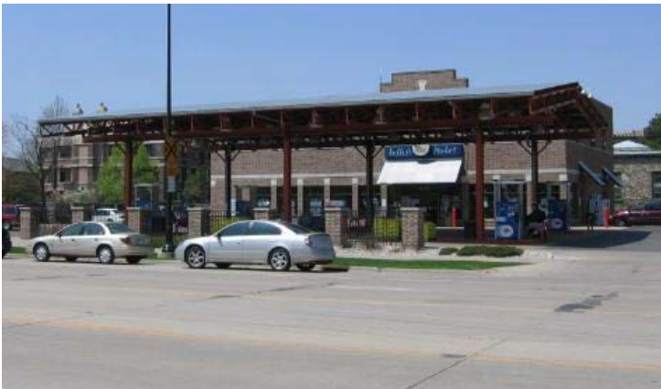
City Assessor’s Office
