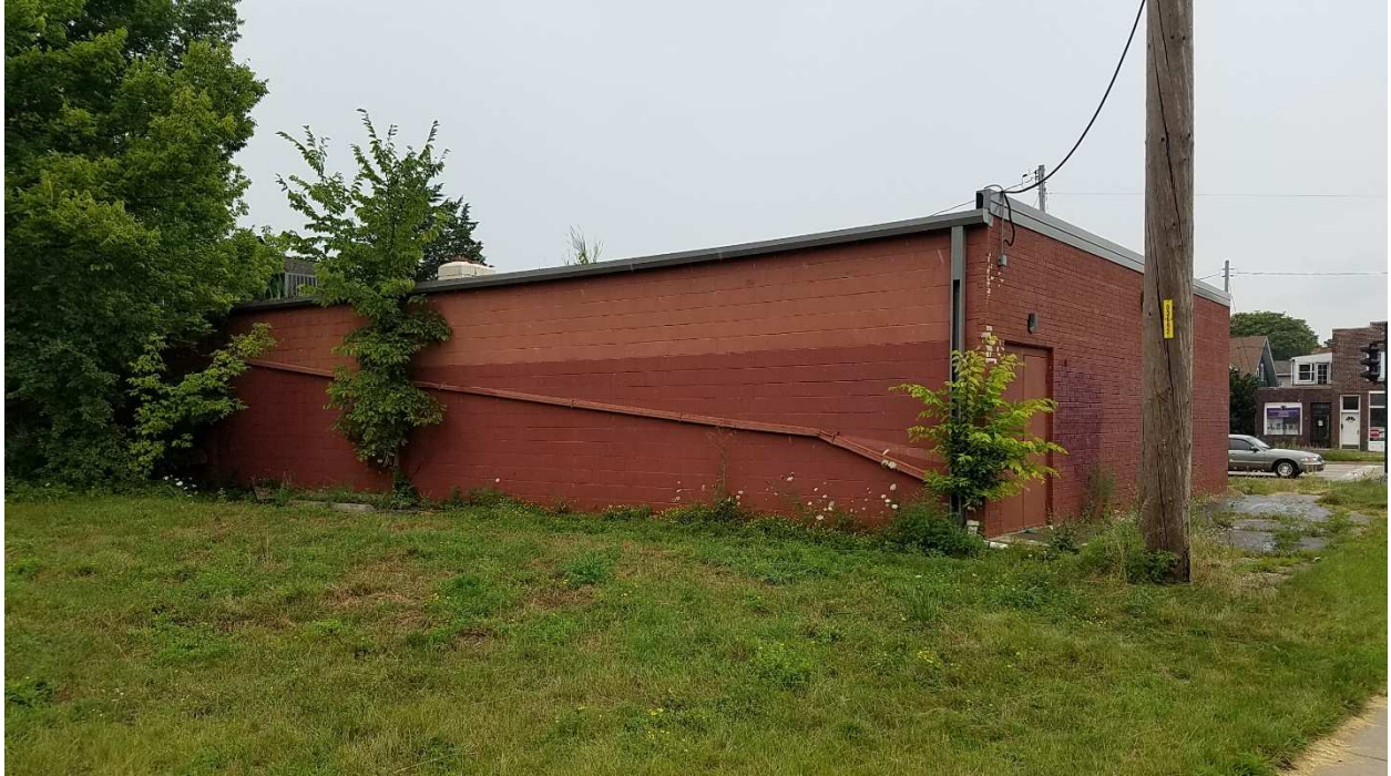
Exterior of commercial building:
