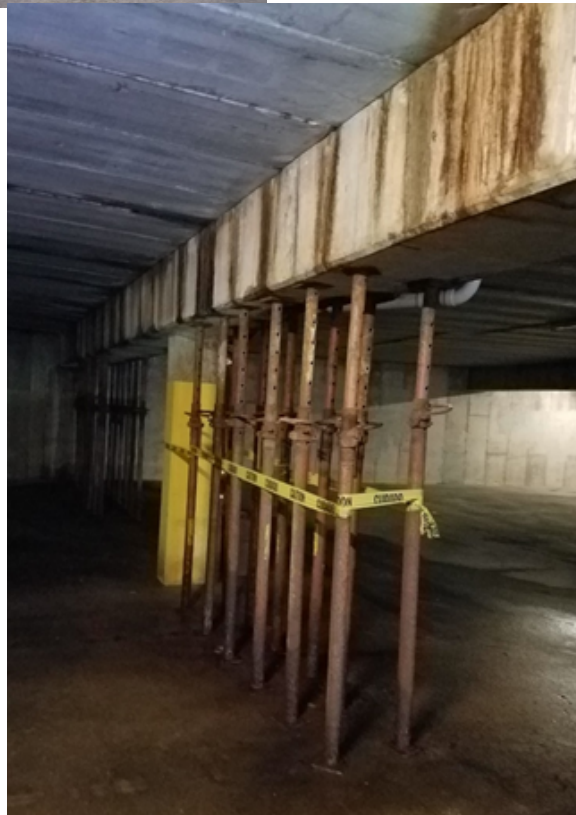
Staining on the concrete beams is from rusted rebar inside the precast concrete planks above and the beams themselves.
