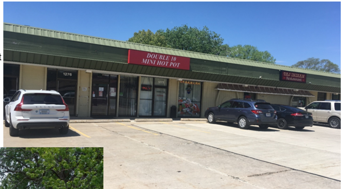
Exterior looking West
