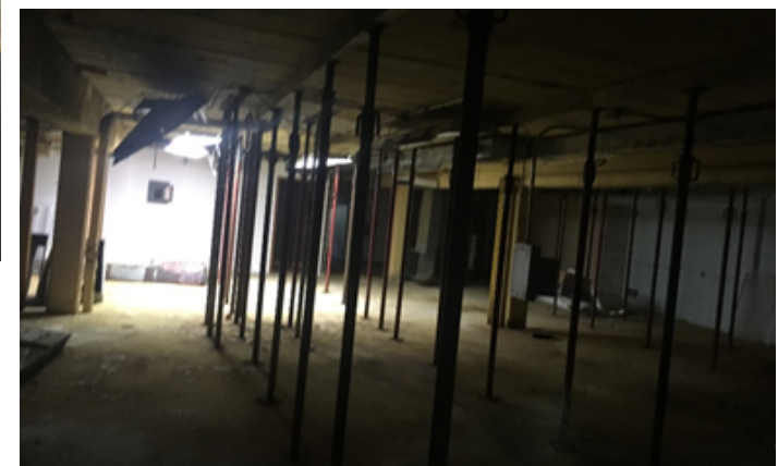
Lower level former office space with temporary shoring posts. Rust staining and spalled concrete visible.
