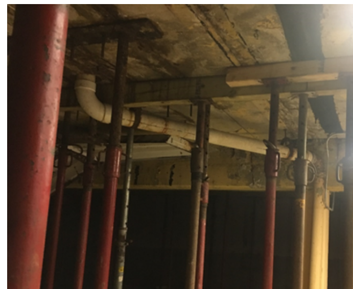
Staining on the concrete beams is from rusted rebar inside the precast concrete planks above and the beams themselves.
