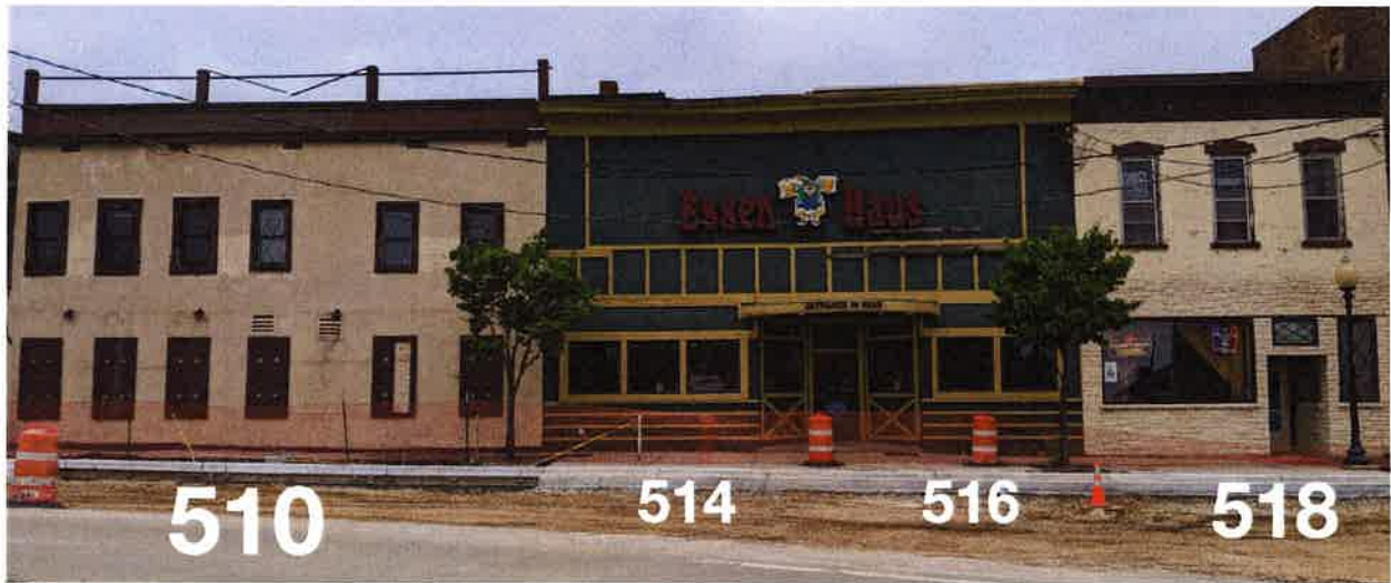
East Wilson Street Facade
