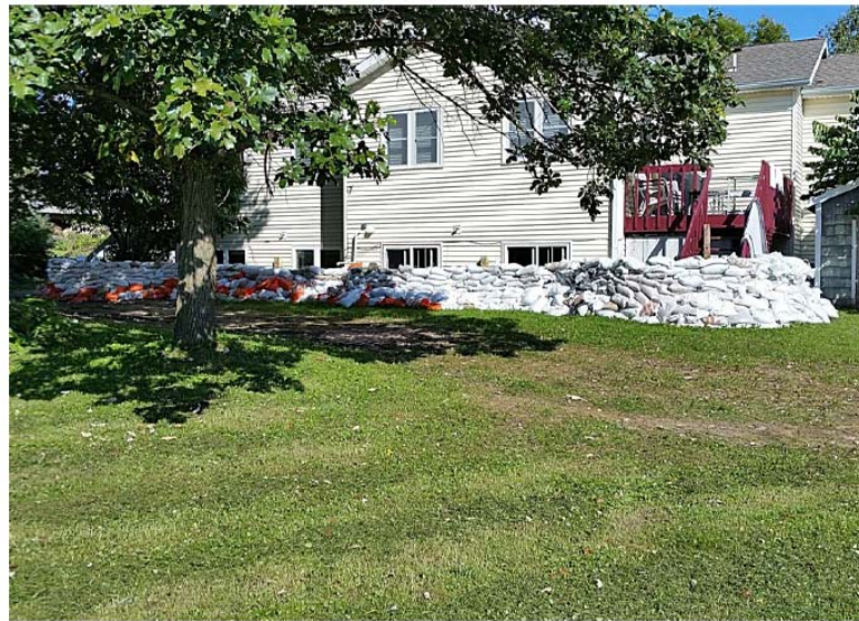
SANDBAGS 3-4FT TALL – SAME HEIGHT AS FLOOD WATERS
