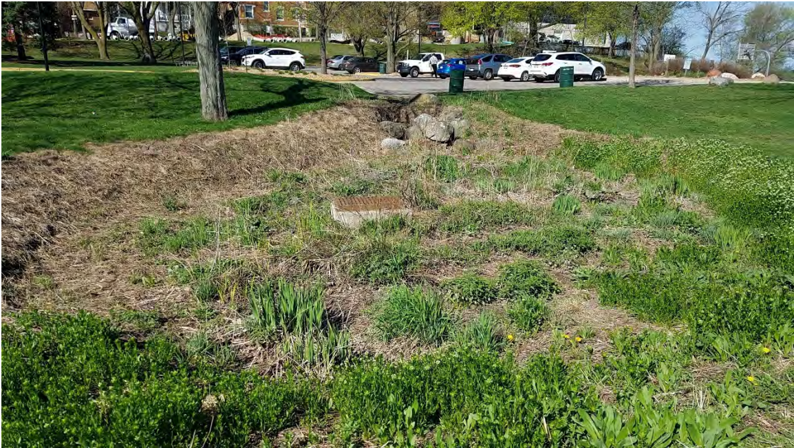
A constructed detention basin contains wetland vegetation.
