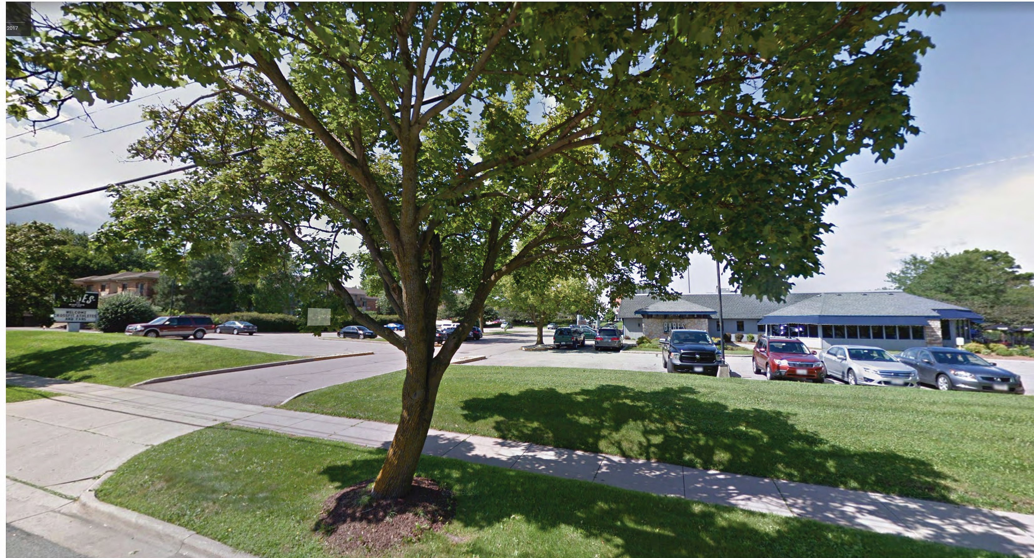
Existing building to be demolished
