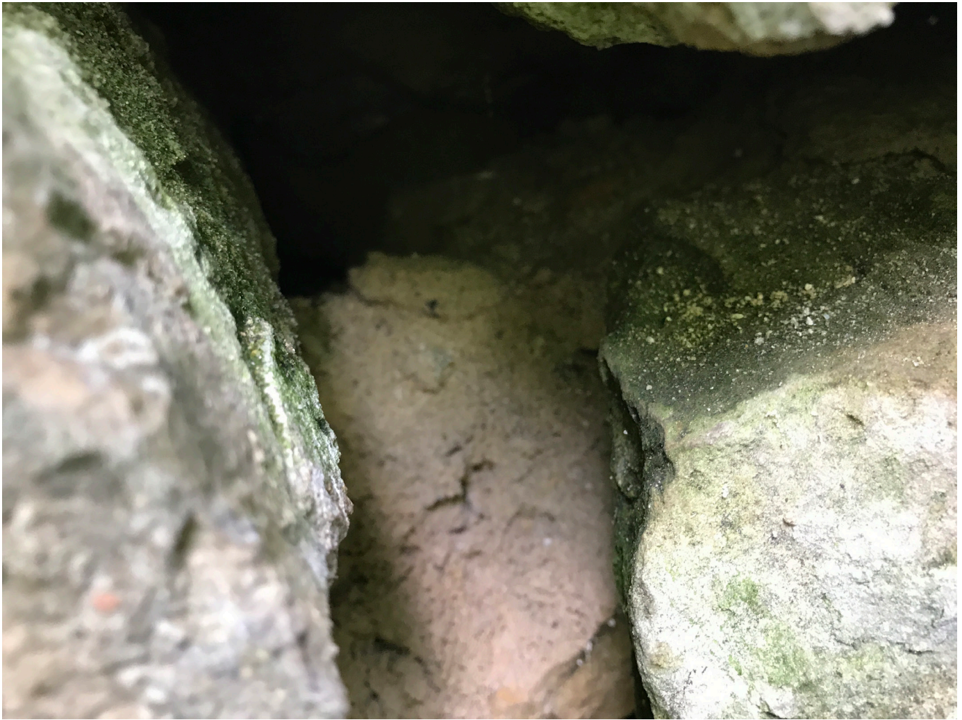
Figure 12: Degradation of the arch stones deeper in the wall is visible from the open joints where the arch has come out of alignment due to settling at the base at the right.
