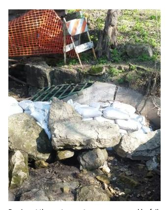
Erosion at the upstream storm sewer caused by failure of the diversion wall
